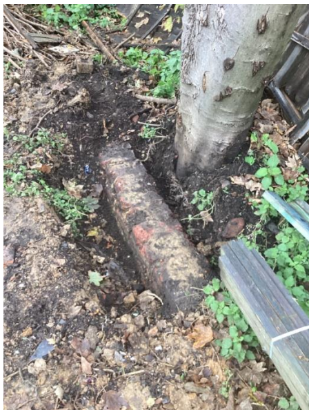
Figure 3.2. Subterranean perimeter retaining wall
