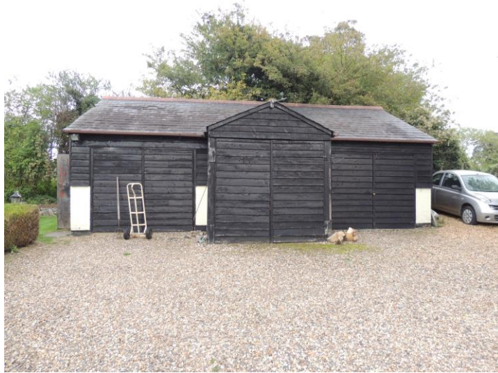
Photo 12: Southern elevation of the workshop
