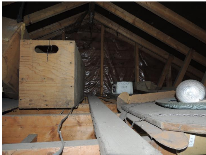
Photo 14: Note lack of evidence of bats in roof space
