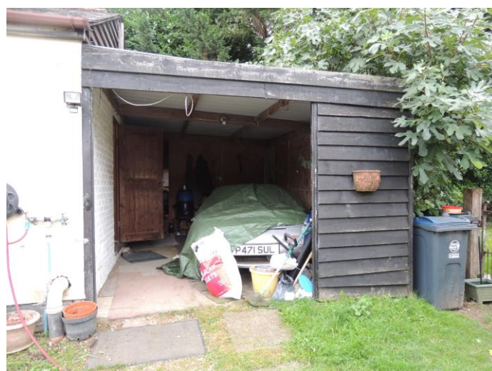
Photo 19: Lean-to car port at the southern end of the building
