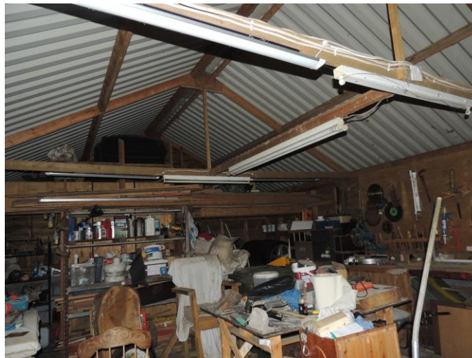
Photo 4: Looking E-W in the shed
