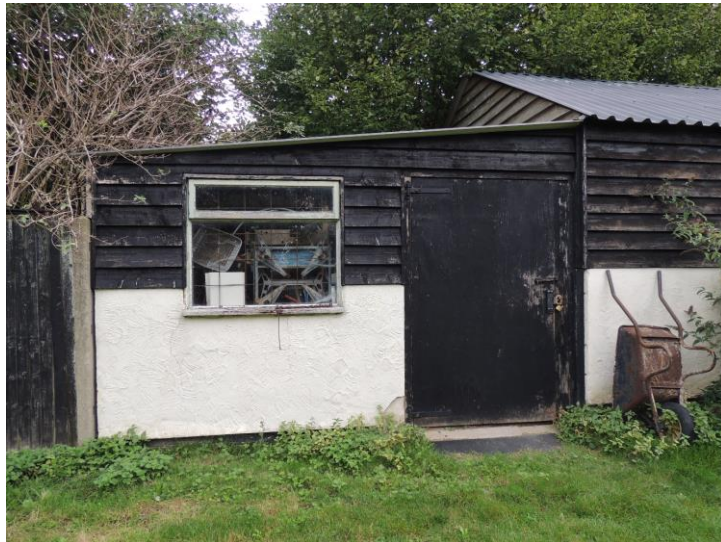
Photo 7: A lean-to store is at the western end
