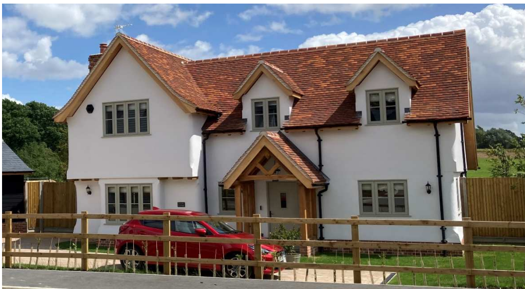
(Elevations of Plot 1 & example of similar house type previously constructed by Pelham Structures Ltd)
