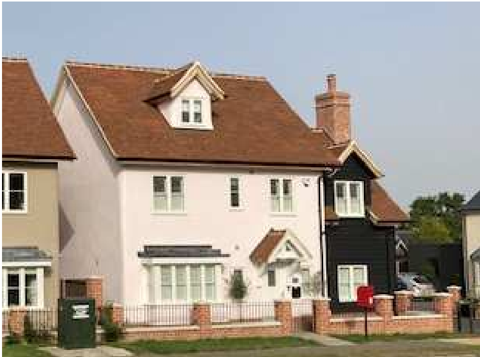
(Elevations of Plots 2/3 & example of similar house type previously constructed by Pelham Structures Ltd)
