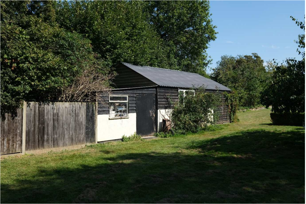
(Garage to be demolished)
