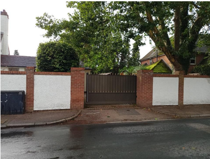
Fig 3. View of existing gates and wall from Duncombe Road. Location of proposed garage clearly obscured from view.
