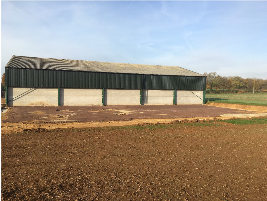
Figure 1: Site before construction.
