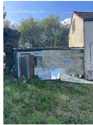
Figure 6. Northern aspect of building D.
