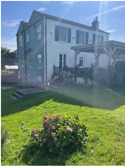
Figure 9. Western aspect of building A.
