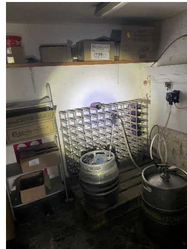
Figure 22. Basement of building A
