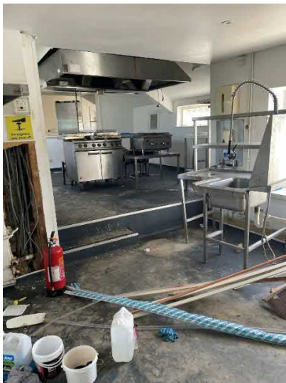
Figure 15. Building A, ground floor kitchen.
