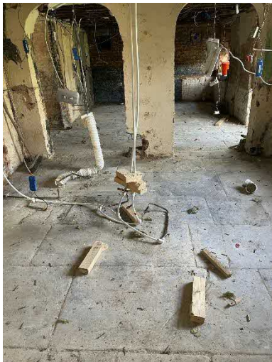
Figure 21. Basement of building A.
