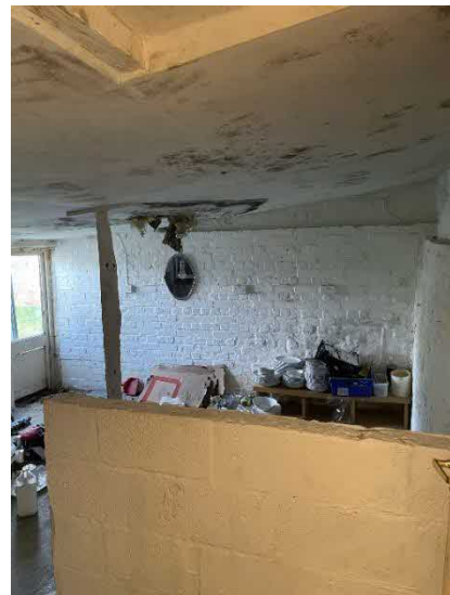
Figure 16. Internal space of building C entered via building A.
