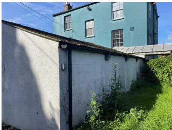
Figure 7. Northern aspect of building B.
