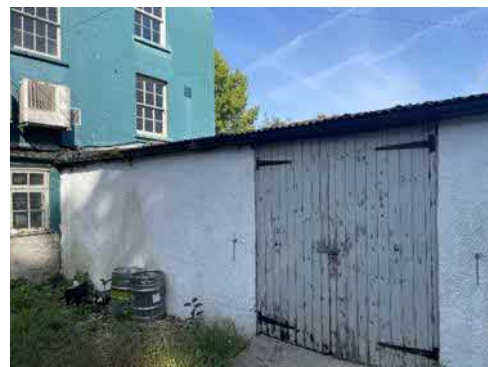
Figure 8. Southern aspect of building B.
