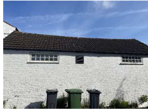
Figure 4. Southern aspect of building C.
