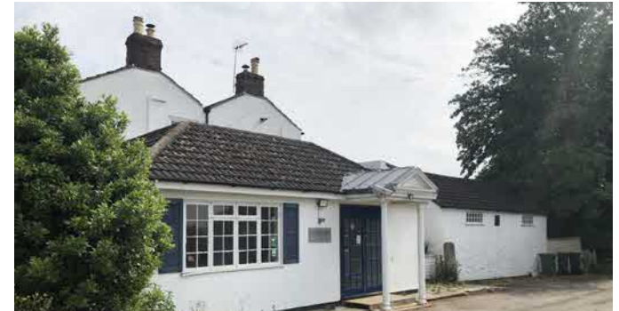
South facing (road) elevation #1
