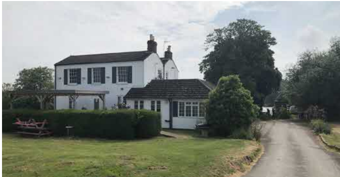
East facing (river) elevation #1
