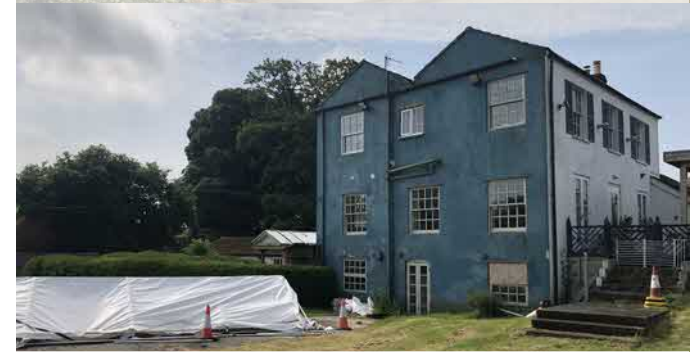
North and east facing elevations #2
