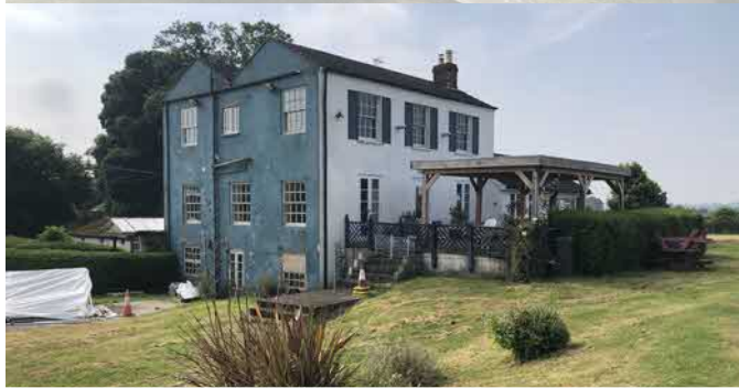
North and east facing elevations #1
