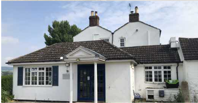
South facing (road) elevation #2
