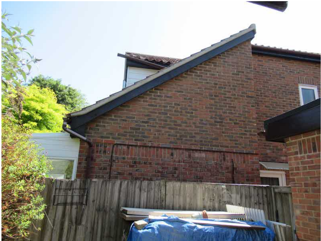
View of No 3 rear extension
