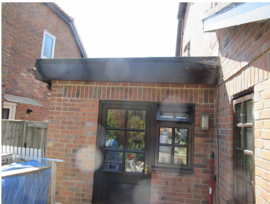
Rear side view adjacent to No 3
