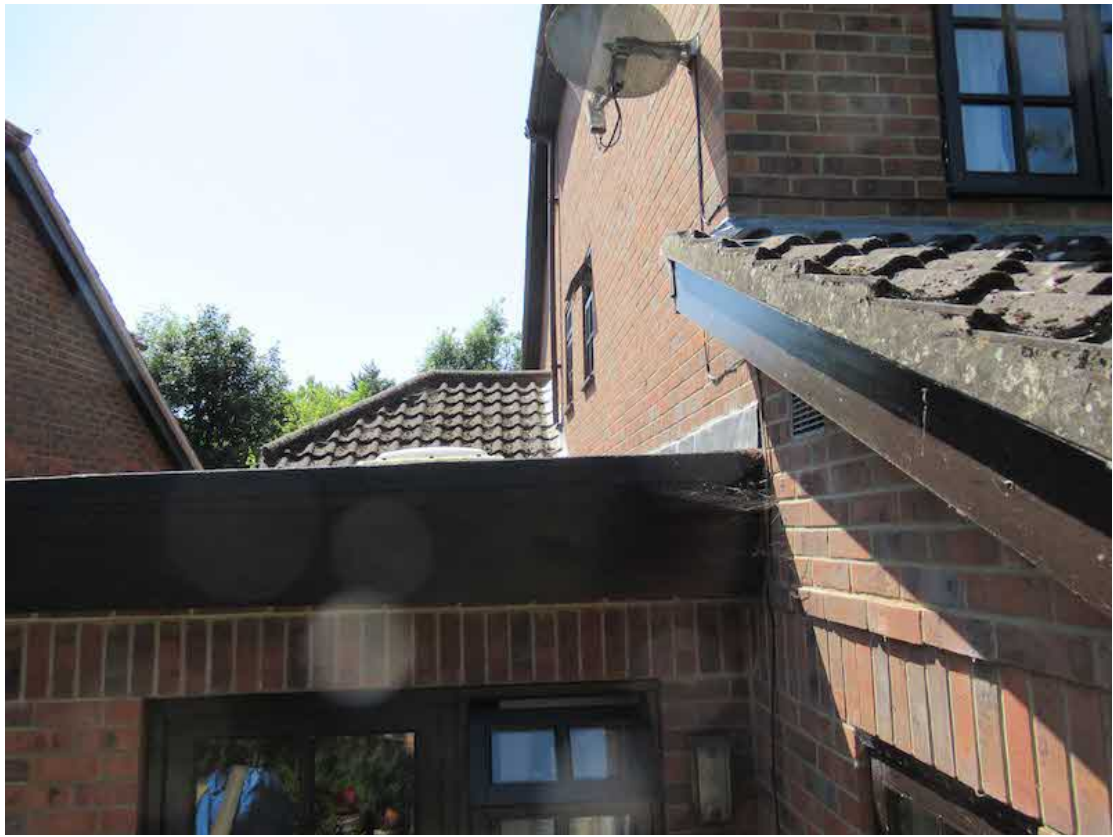
View of 1st floor adjacent to No 3
