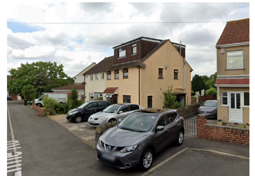
Figure 10: View of flat roof dormer windows to front and rear of 23 Lime Road (Obtained from Google Earth, October 2023)
