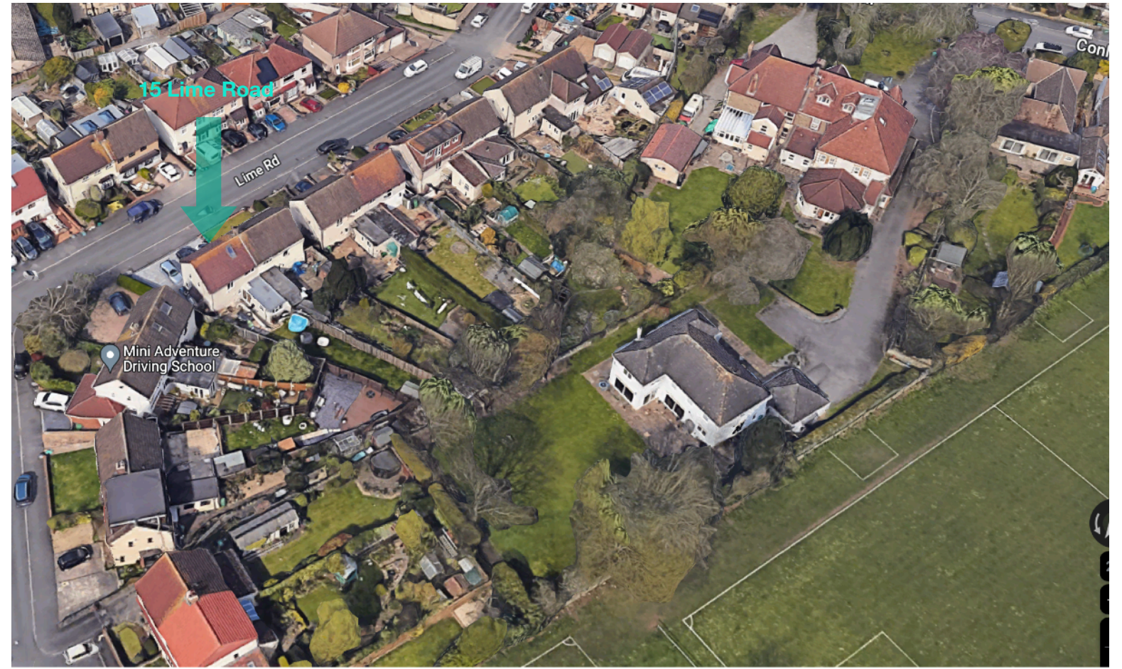
Figure 2: Aerial view from South East show rear of 15 Lime Road - labelled (Obtained from Google Earth October 2023)
