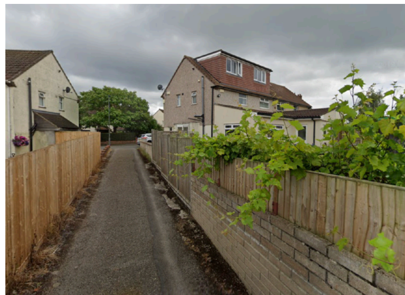
Figure 9: View of flat roof dormer to rear of 22 Lime Road from public lane (Obtained from Google Earth, October 2023)
