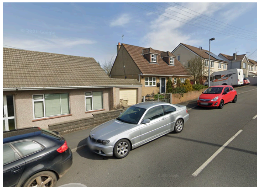
Figure 8: View of traditional dormer windows to front of 21 Conham Hill (Obtained from Google Earth, October 2023)
