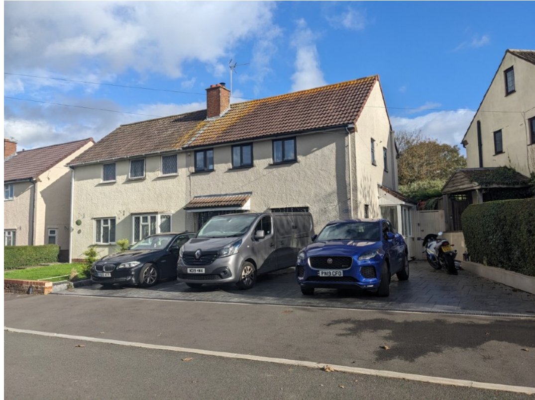
Figure 4: View of front of house (October 2023)
