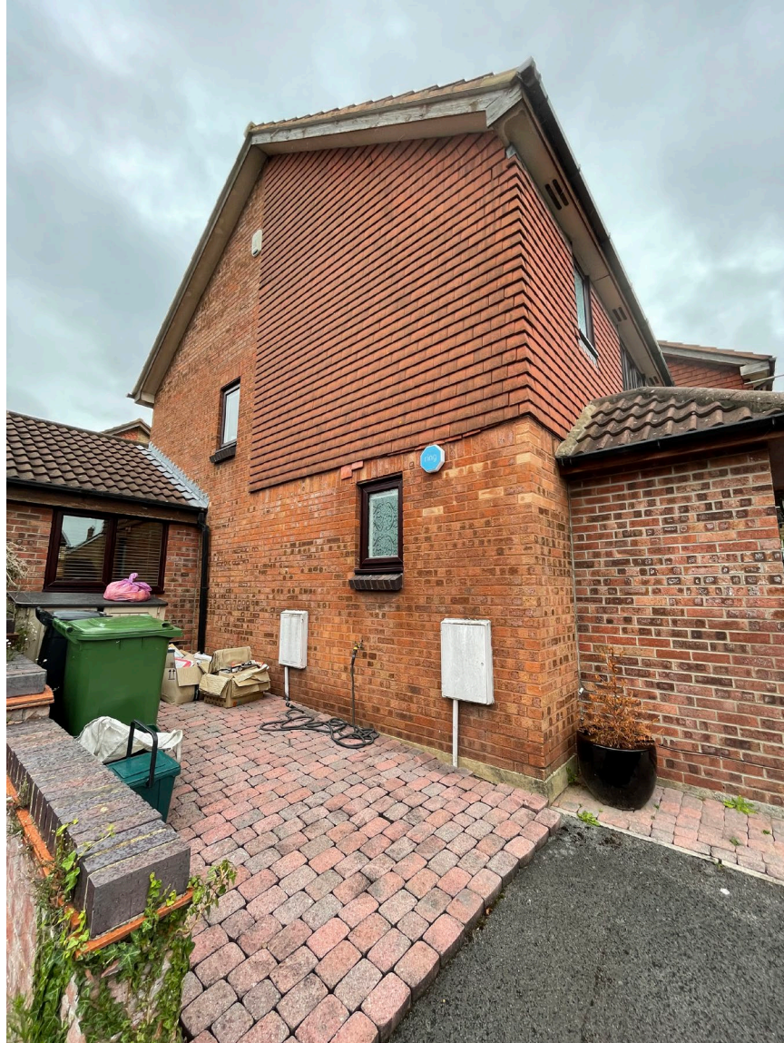
Fig. 2 – Side elevation of property.
