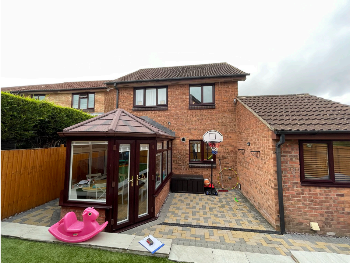
Fig. 3 – Rear Elevation of property.
