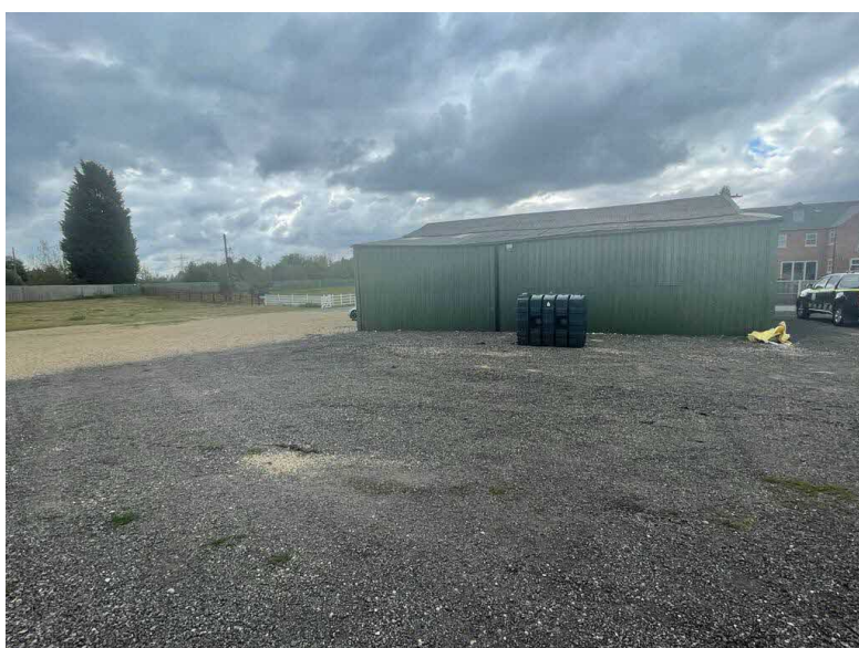
Existing metal Cladded store on site with concrete floor.
