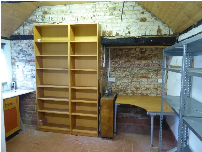
Figure 24: View of attached outbuilding at west of main pile
