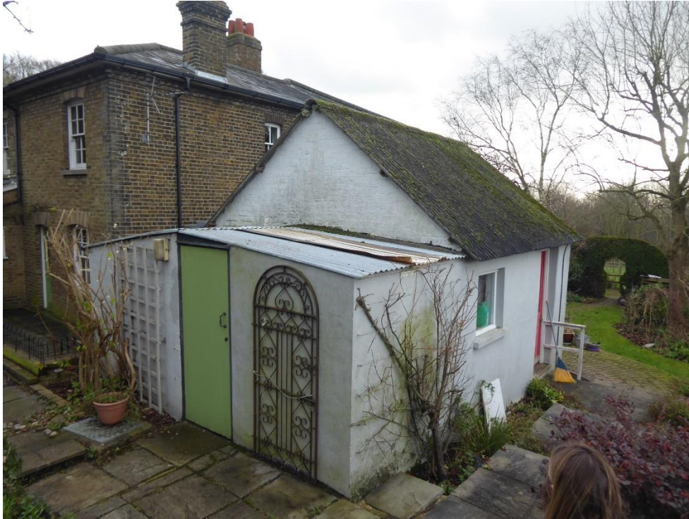
Figure 19: View of north west corner of outbuilding
