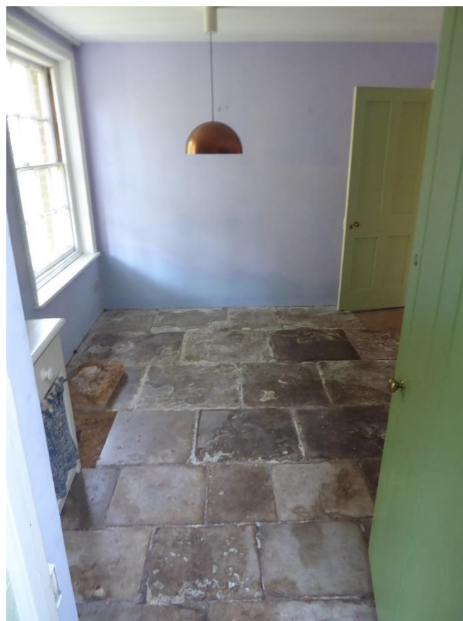
Figure 23: View of original kitchen at northeast corner
