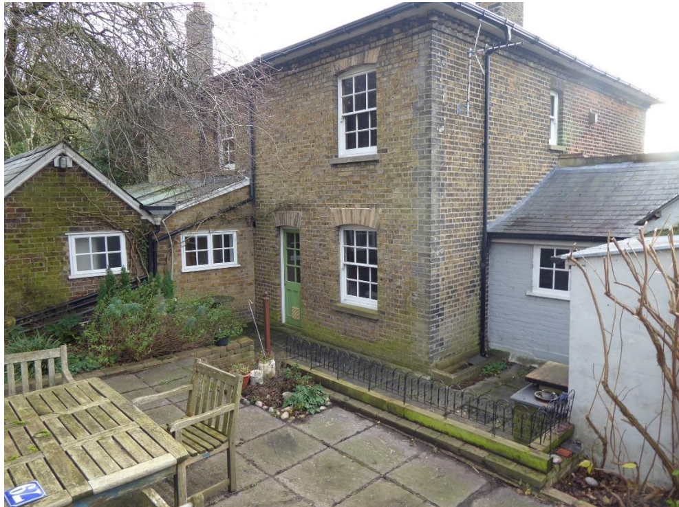
Figure 17: View of northwest corner
