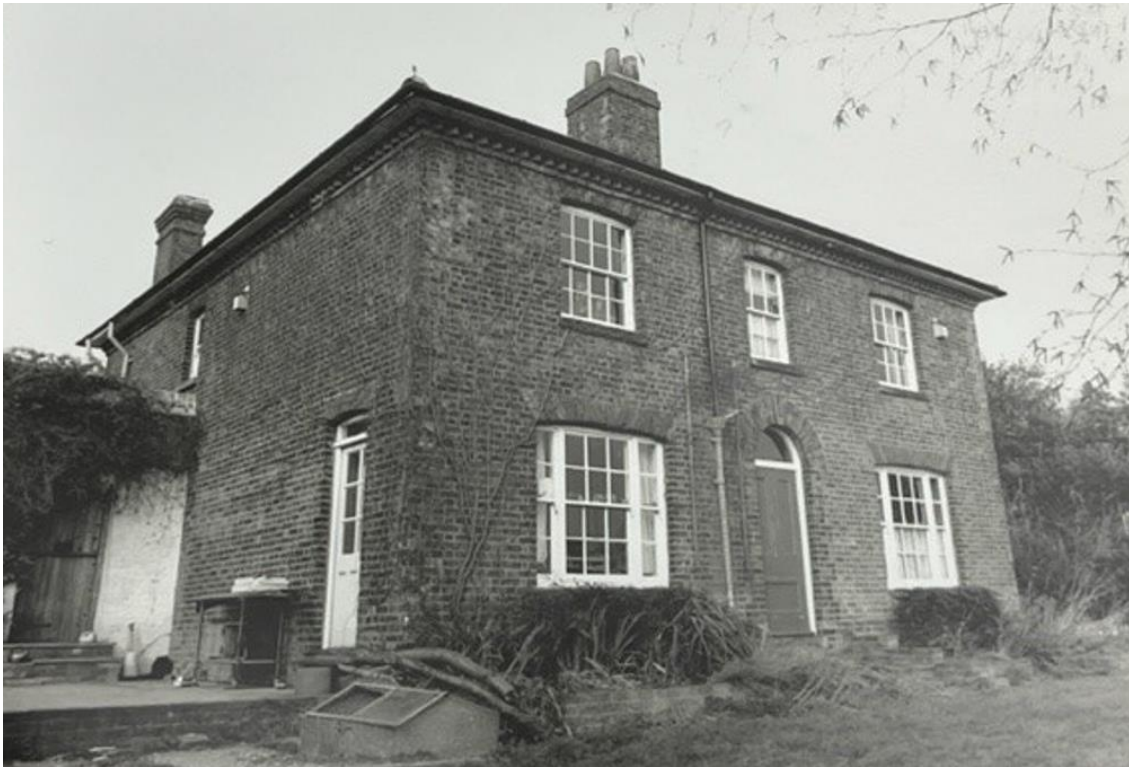
Figure 12: Photograph of Pump Farmhouse from southwest, 1990 (Essex County Council)
