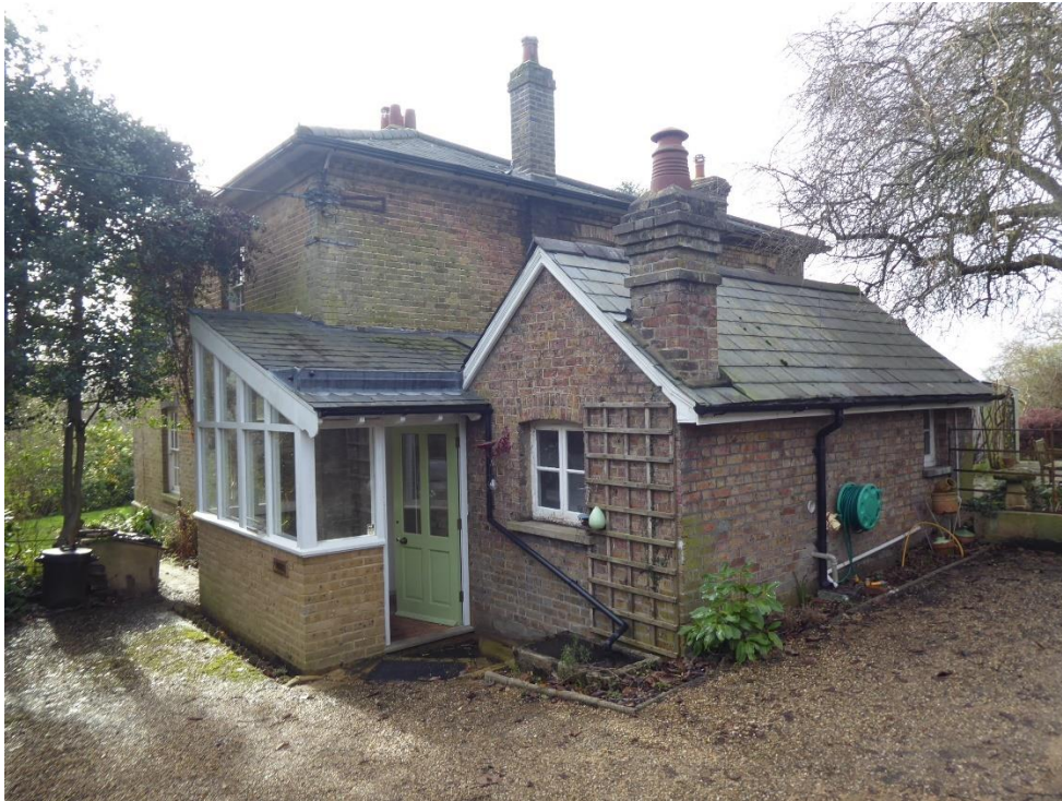
Figure 16: View of northeast corner
