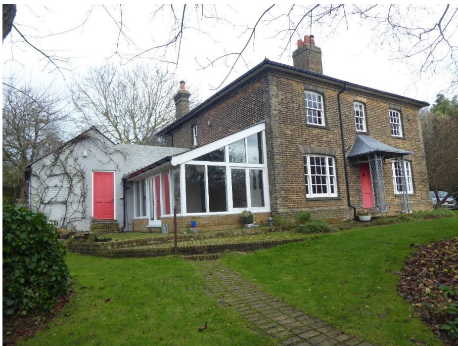
Figure 18: View of southwest corner
