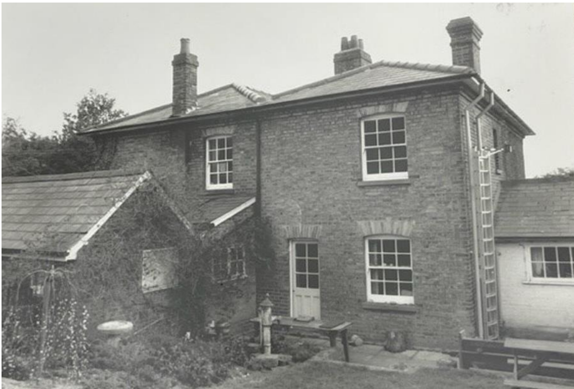
Figure 13: Photograph of Pump Farmhouse from north, 1990 (Essex County Council)
