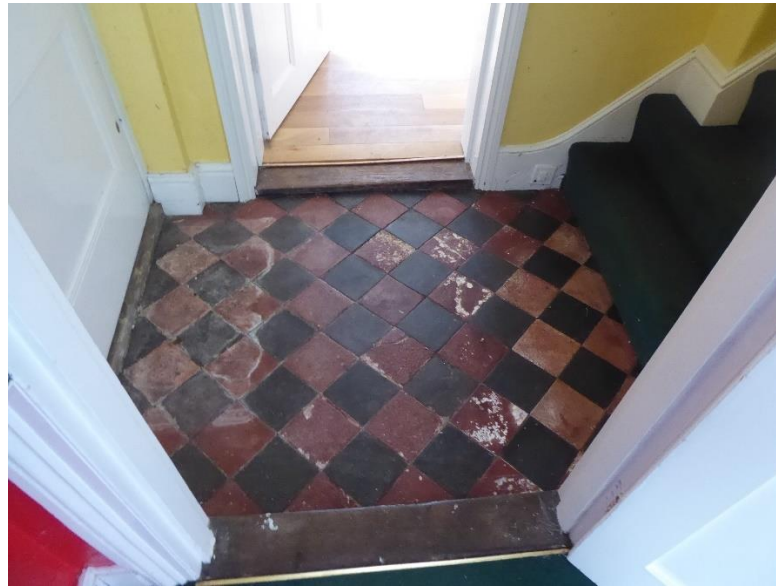
Figure 26: View of lobby to main entrance with early tiles
