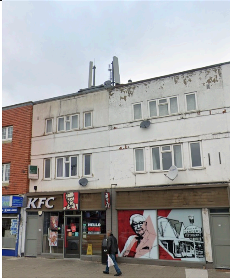
Image 1c: The Existing Site
