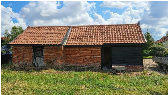
Photo 3 North section west elevation showing door with gap above door - and new roof and fascia boards
