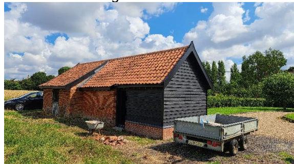
Photo 4 North elevation - new barge boards and re-pointed mortar work
