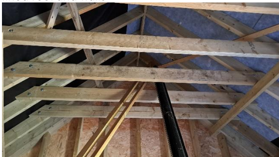
Photo 11 South section - timber frame structure and lined roof and walls
