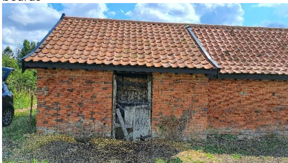
Photo 3 North section west elevation showing door with gap above door - and new roof and fascia boards
