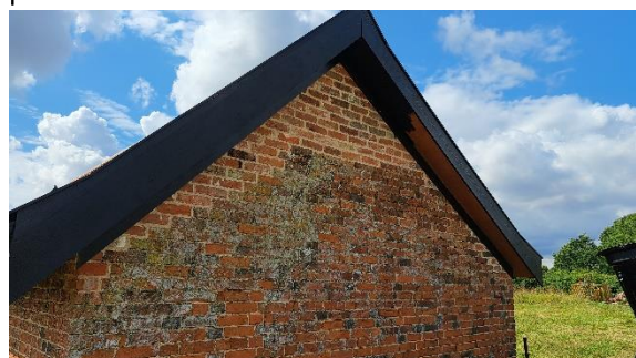
Photo 4 North elevation - new barge boards and re-pointed mortar work
