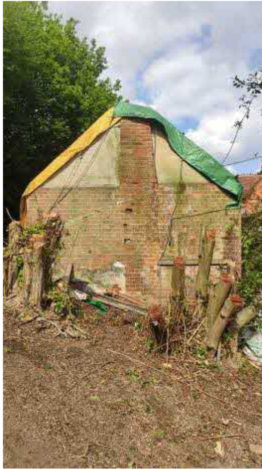
Photograph 19 – External view of south facing gable.
