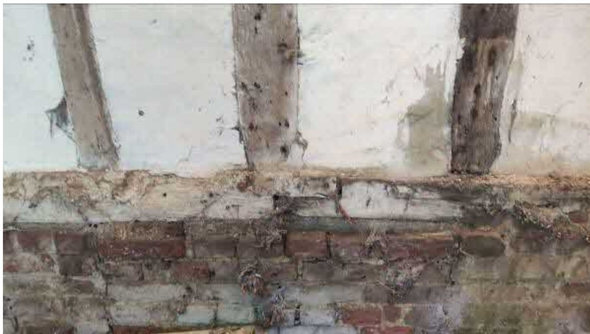
Photograph 17 – Bottom wall plate on west side showing the half lapped joint.
