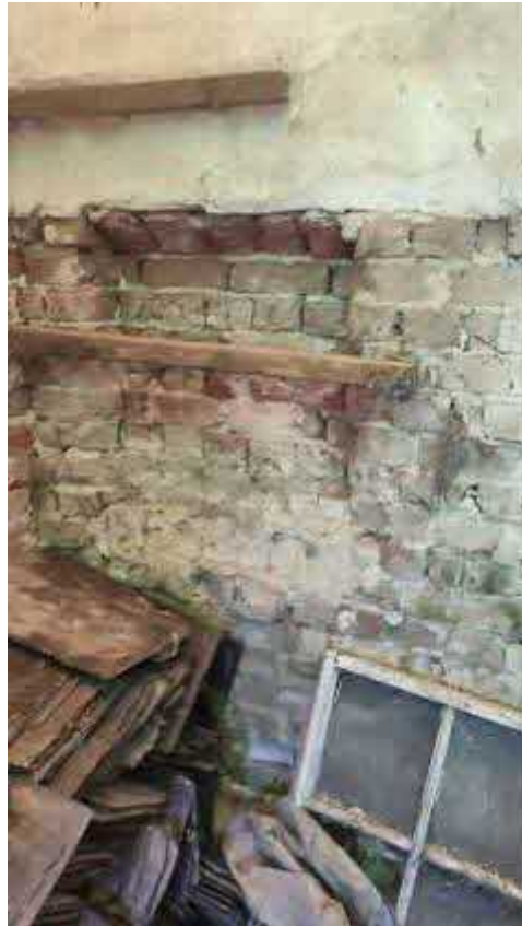
Photograph 15 – Pocket cut into the brick wall on the west facing elevation.
