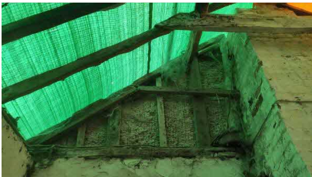
Photograph 10 – Left hand spandrel panel at the south gable.
