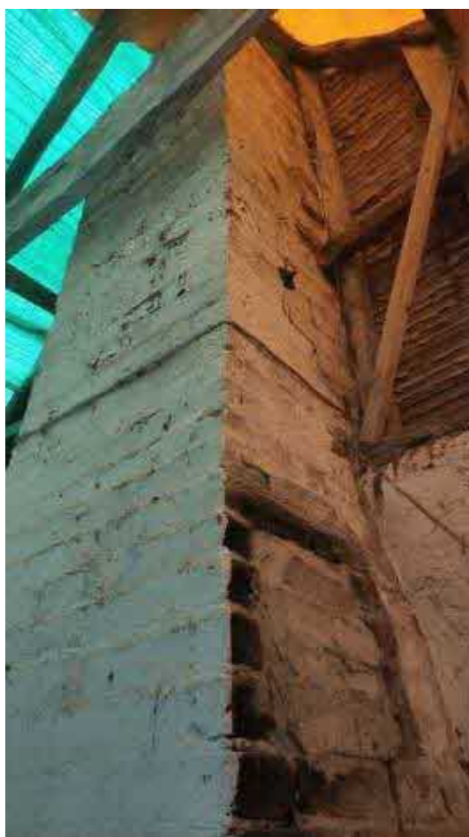
Photograph 12 – Existing steel tie through the stack at the south end.
