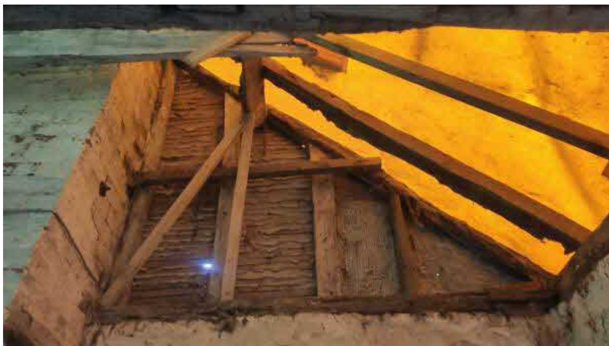
Photograph 11 – Right hand spandrel panel at the south gable.
