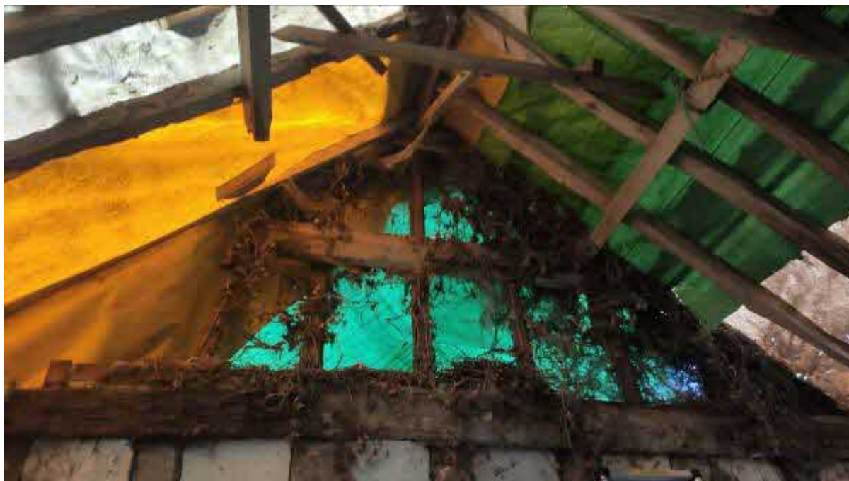
Photograph 05 – Spandrel panel at the north end.
