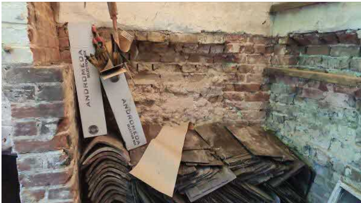
Photograph 14 – Pocket cut into the south gable wall.
