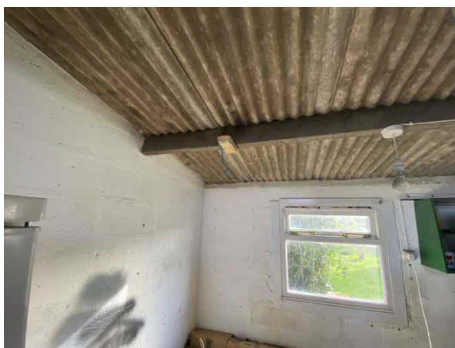
Figure 5. Underside of the roof.
