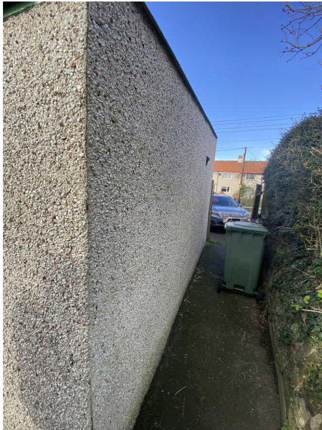
Figure 3. The east wall of the garage
