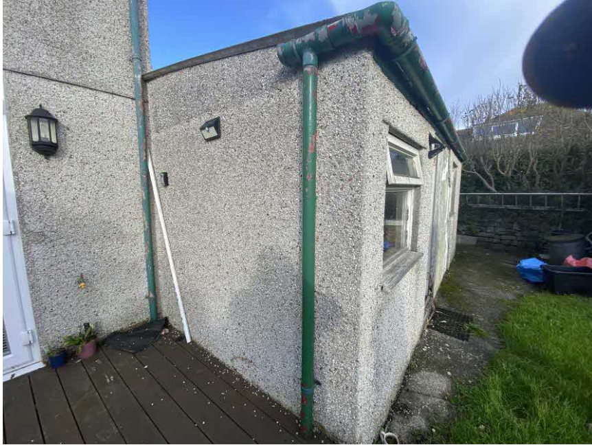
Figure 2. The south end of the garage.
