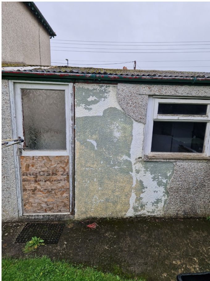
External rear southern wall showing no gaps or crevices around doors or window frames
