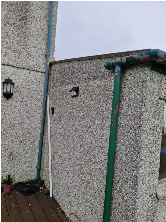
Rear side external western wall clearly showing no gaps or crevices
