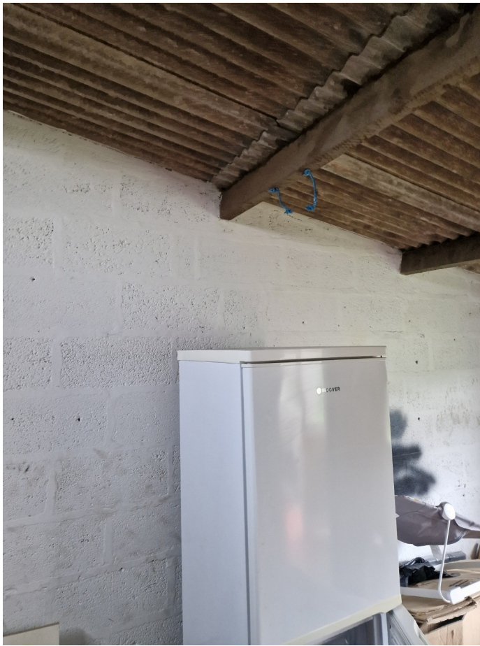
Internal eastern gable wall and window showing no gaps or crevices
