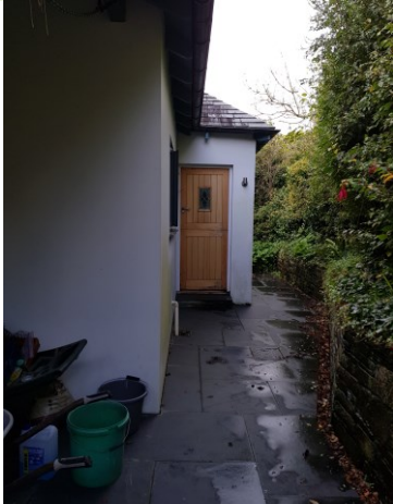
Aspect where extension will be constructed.
