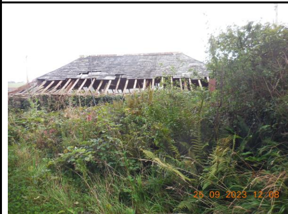
Plate 5. The northern elevation of the barn
