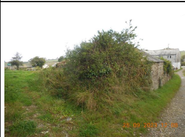
Plate 6. The southern track and southern wall of the barn
