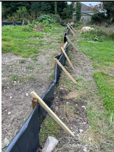
Plate 13. Reptile translocation fencing
