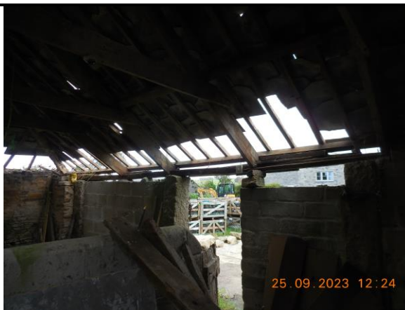
Plate 11. The internal eastern wall of the barn
