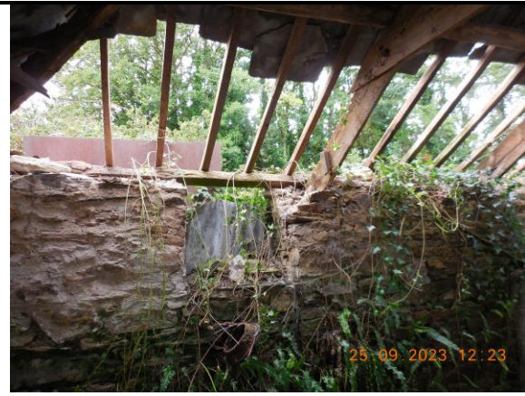
Plate 10. The internal northern wall of the barn
