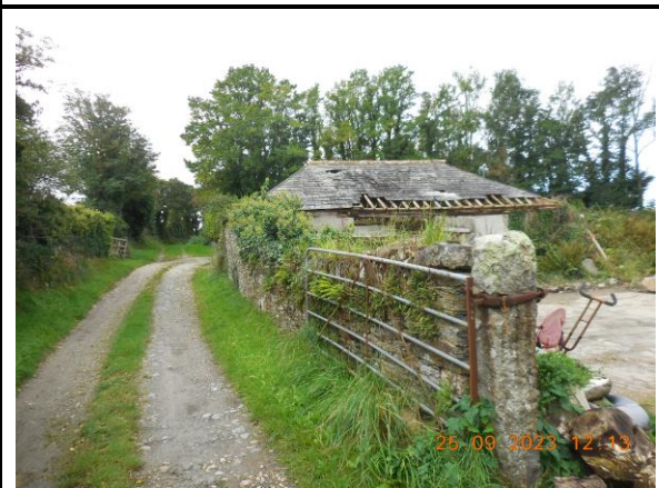
Plate 8. The eastern aspect of the barn and southern track
