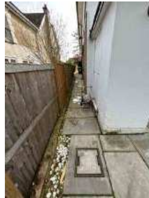
MH1 to MH2
