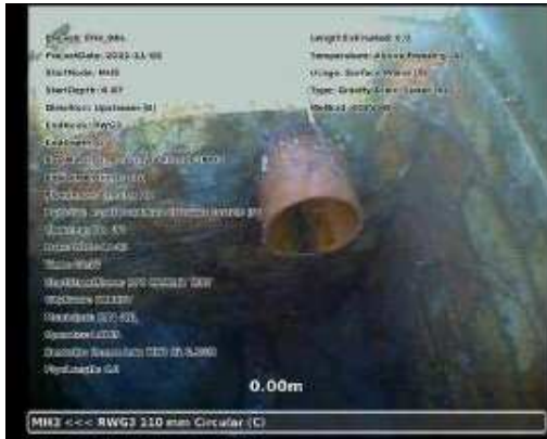
20221102-092841-snap0000.jpg, 00:00:00, 0.00 m Start node, manhole, reference: MH3
