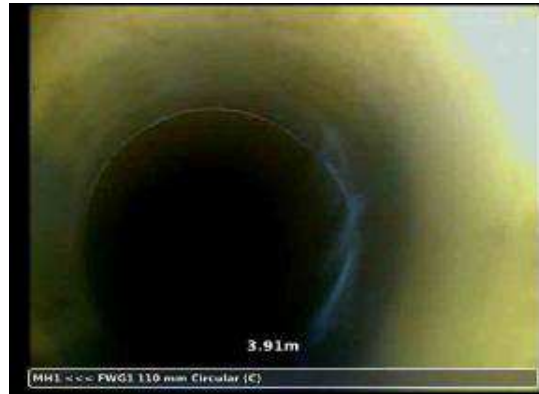
FWG1X_d1f31eae-14be-428c-b6e3-6148890389bb_20221103_101340_409.jpg, 00:00:21, 3.91 m General photograph taken at this point
