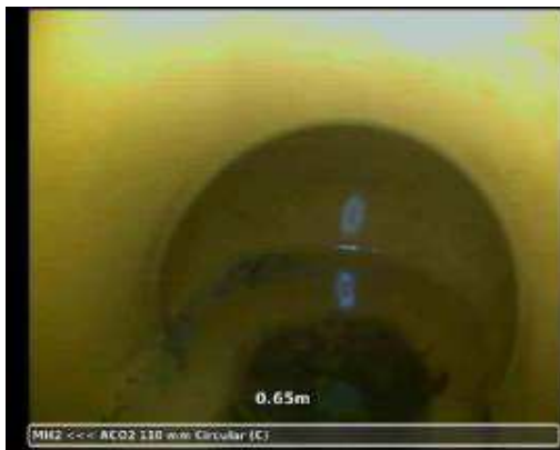
20221102-091807-snap0003.jpg, 00:00:17, 0.65 m Finish node, gully, reference: ACO2
