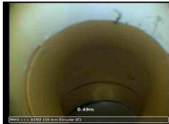
ACO2X_7dc139ce-aeb6-4b22-838a-7008bf17a777_20221103_102550_845.jpg, 00:00:10, 0.49 m Line deviates down
