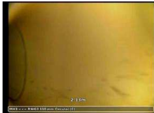
RWG3X_5cb0c9bf-0b0f-48bd-9de4-727545d8e9e1_20221103_103442_854.jpg, 00:00:13, 2,13 m Line deviates left
