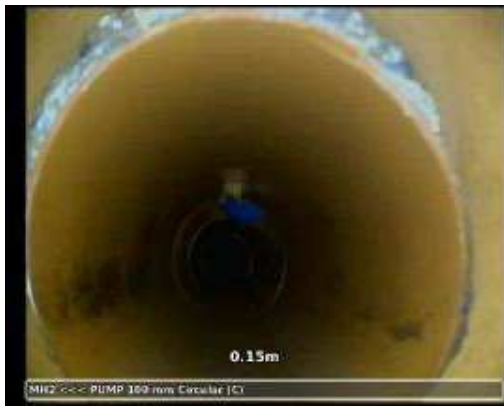
20221102-090846-snap0001.jpg, 00:00:11, 0.15 m Material changes to polyvinyl chloride, 110
