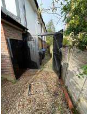
MH3 to MH2
