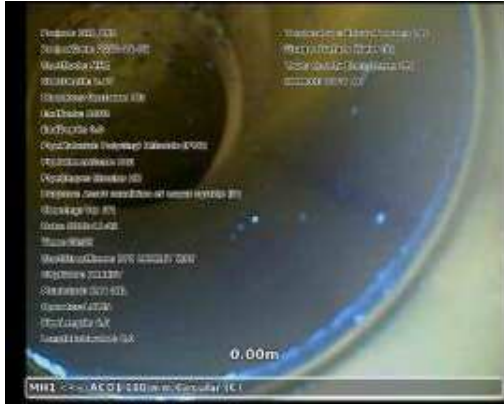
20221102-083010-snap0000.jpg, 00:00:00, 0.00 m Start node, manhole, reference: MH1
