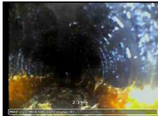
MH2X_0c38dde7-d8bb-4f88-8d2b-98dfbd033046_20221103_102754_779.jpg, 00:00:32, 2.39 m General photograph taken at this point
