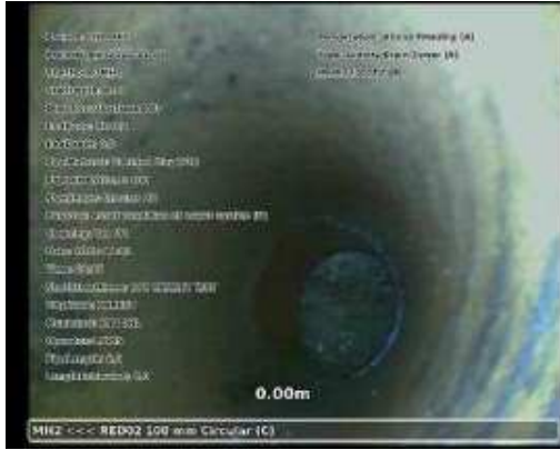
20221102-091350-snap0000.jpg, 00:00:00, 0.00 m Start node, manhole, reference: MH2
