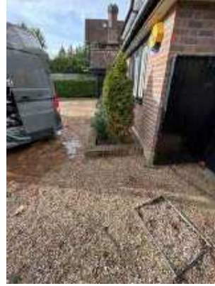
MH3 to MH4
