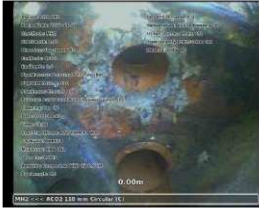
20221102-091807-snap0000.jpg, 00:00:00, 0.00 m Start node, manhole, reference: MH2
