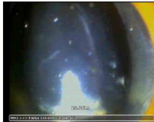
20221102-083127-snap0001.jpg, 00:00:50, 10.26 m Finish node, gully, reference: FWG1
