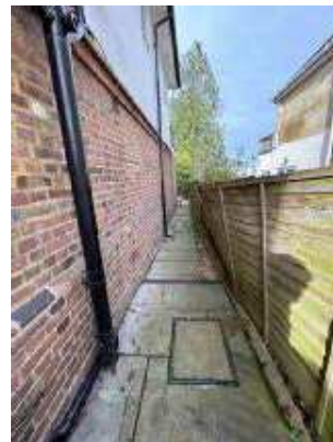
MH2 to MH1
