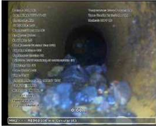
20221102-091424-snap0000.jpg, 00:00:00, 0.00 m Start node, manhole, reference: MH2
