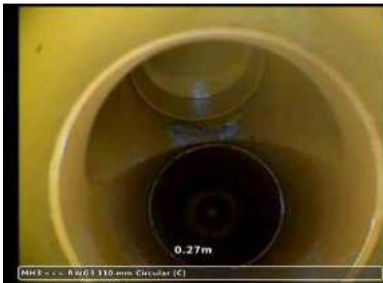
RWG3X_cf47935a-85fd-4da2-a48d-ed589d96b3f2_20221103_103426_234.jpg, 00:00:06, 0,27 m Junction at 12 o'clock, diameter: 110mm, Capped
