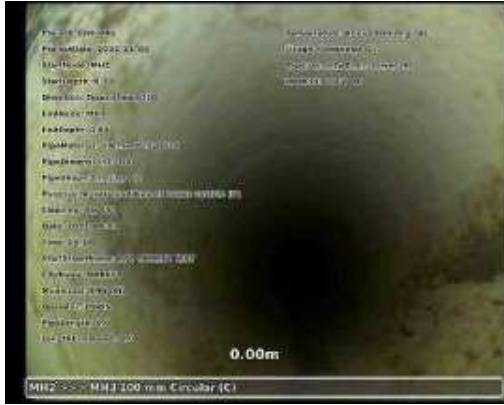
20221102-092005-snap0000.jpg, 00:00:00, 0.00 m Start node, manhole, reference: MH2
