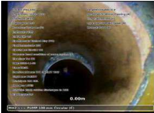
PUMPX_47a25daf-bdea-421f-a2b7-49eb1da782b4_20221109_151411_483.jpg, 00:00:00, 0.00 m Start node, manhole, reference: MH2
