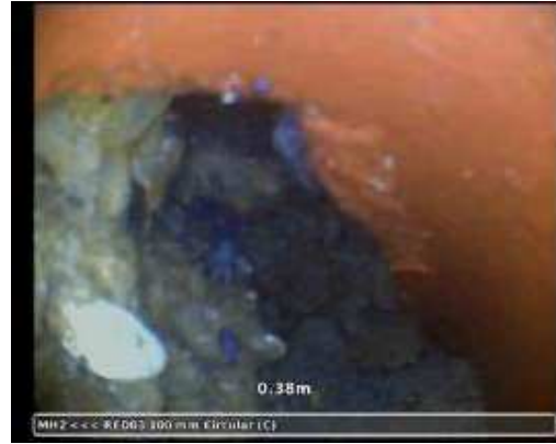
20221102-091424-snap0001.jpg, 00:00:09, 0.38 m Finish node, major connection without manhole, reference: RED03
