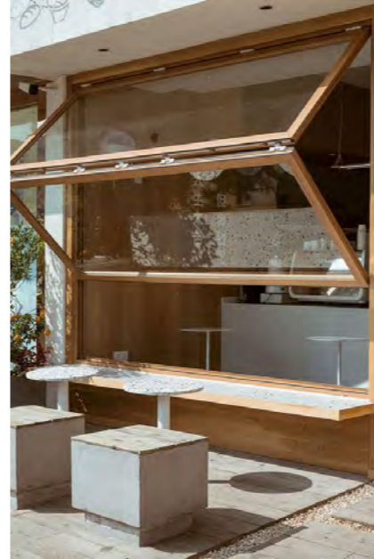
Timber (Accoya) bi-fold service hatch
