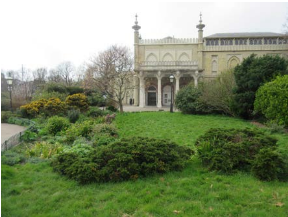
View 7, west to Museum and entrance, formerly (from 1900) to the Dome.
