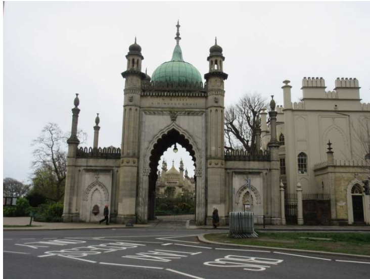
View 1a, south through North Gate to Porte Cochere.
