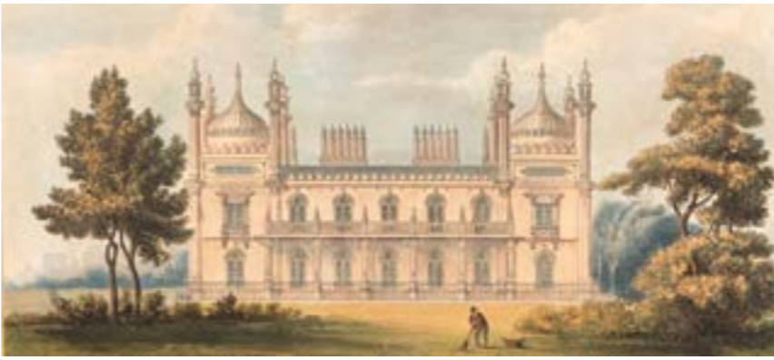
This view is similar to the layout on the ground plan. The sea view is visible far left.
