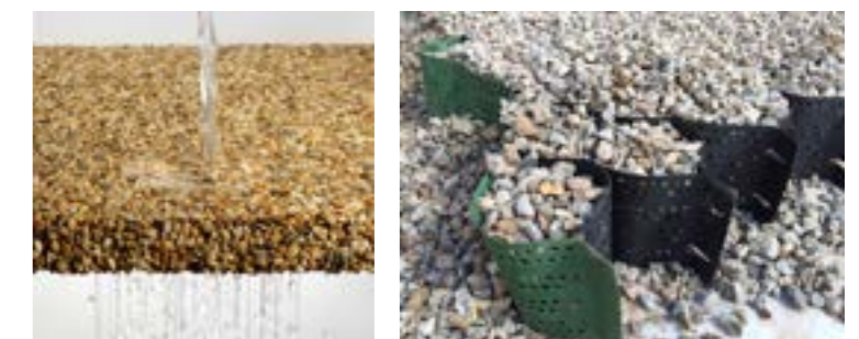
Resin bound gravel & CellWeb sub base detail
