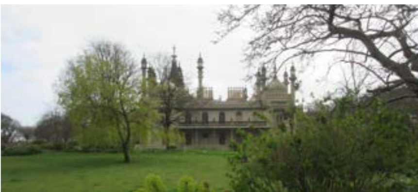
The two trees require removal. The sea view is obscured by trees, but not irreversible.
