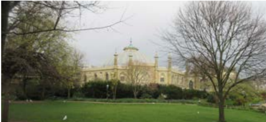
This view is taken from slightly further away. The tower block rises above the tent roof of the Music Room.
