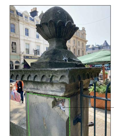
Existing pier. Replace stone panel in matching stonework. Allow for associated repairs to exposed brickwork using lime mortar. Provide sample of stone for approval.
