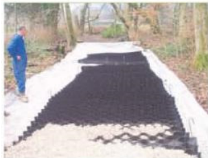
CellWeb during installation.
