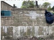
4.3 Investigation of existing foundations to piers adjacent to heavily planted areas to the Old Stein to the east of the site to investigate cause of large horizontal cracks and damaged finish (allow for 3 no. locations to the northeast of the site where existing ground levels vary the most). See drawing P1154-RHP-ZZ-00-DR-A-1000 for details of locations to be agreed on site.
