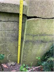
4.4 McLaren Boundary wall cracked balustrade to East Lawn. Samples of the concrete be required to determine its composition to inform a suitable repair strategy. A specialist should be approached to carry out this sample analysis and suitable locations agreed on site (allow for 2 no. locations to the east lawn where significant cracks can be observed to the piers by the ornamental ponds). See drawing P1154-RHP-ZZ-00-DR-A-1000 for details of locations to be agreed on site.
