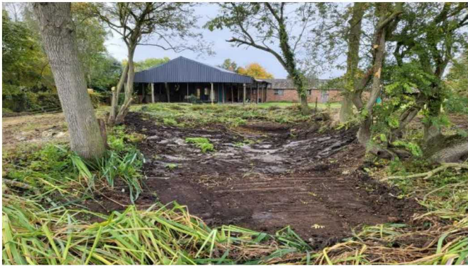
Pond after works.
