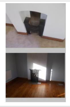
Material Comments: Theses photos were taken due to no access to the live cast pipes to fireplaces in areas 3 & 7 these were both presumed to contain asbestos until further inspections.
