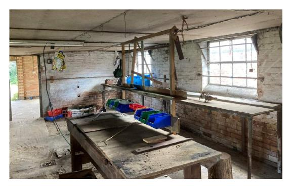
There was efflorescence noted in the top right corner of the interior wall, the extent of the efflorescence internally is hard to gauge due to the previous lime wash, also some holes had been cut in this wall.
