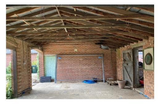
There is a 440mm thick brickwork pier abutting the return wall to the barn has no evident toothing. The junction at the other end of the wall where it abuts Garage 2 shows vertical cracking and signs of previous repairs.
