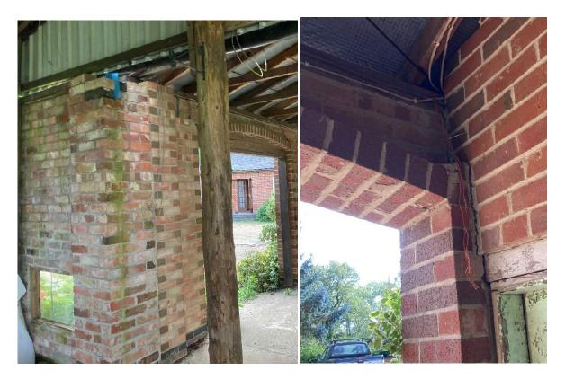
The lintels over the garage door openings show signs of movement with vertical and diagonal cracking with previous mortar repairs. There was no evidence of lintels over these openings other than the brickwork bonding.
