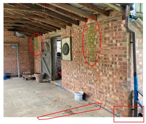
The ground floor slab is 120mm thick unreinforced concrete on blue polythene on 180mm fill on clay. There is a fine crack to the full length, see above.
