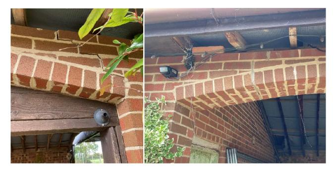
To the external wall of Workshop 2, that forms an internal wall to the garage, there are a couple of areas of mossstained masonry and the is a single cracked brick to the lower corner adjacent the downpipe and gully.
