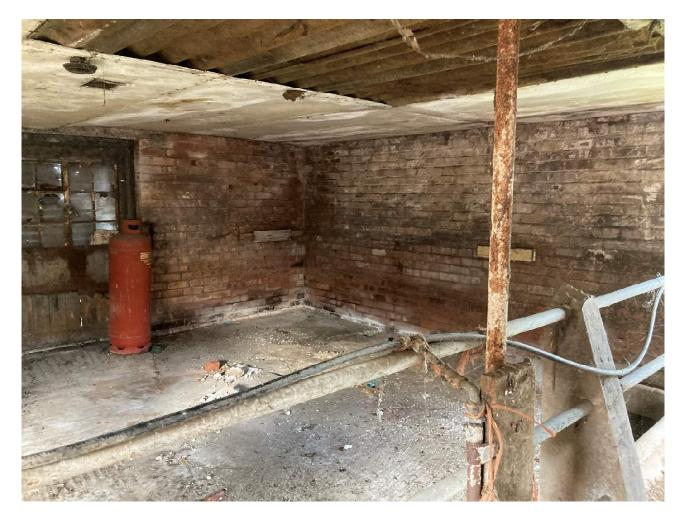
There was efflorescence noted in the top right corner on the inside face of the exterior wall, the extent of the efflorescence internally is hard to gauge due to the previous lime wash.
