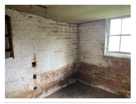
The concrete slab was 100mm thick on white polythene on 125mm crushed brick fill. The slab was in poor condition due to its previous use with level changes, steps and chases where it appears that brick piers have been removed in the past.
