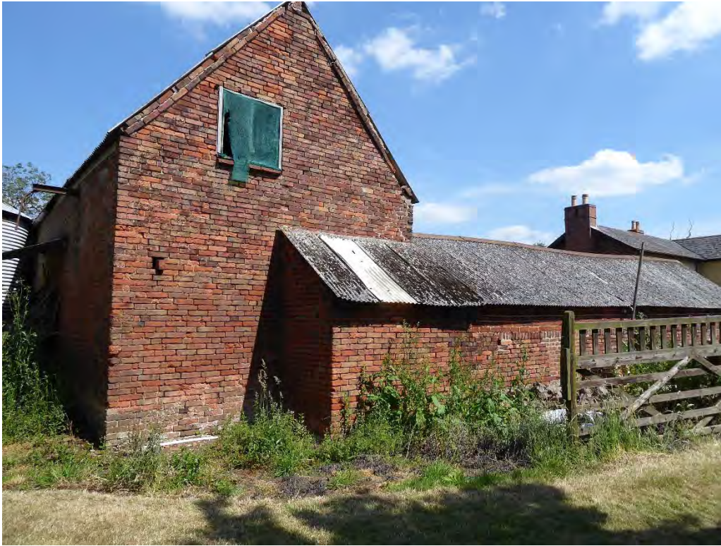
Plate 13: Steep asbestos roofed barn and single storey asbestos roofed byres, viewed south
