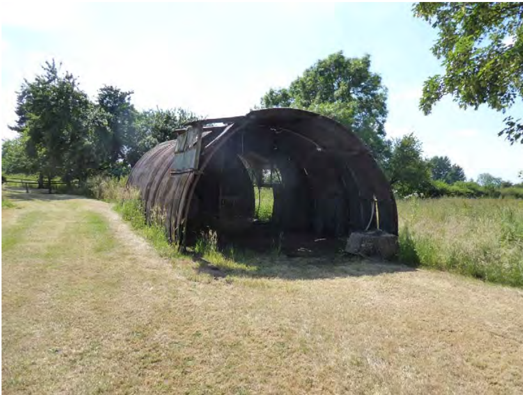
Plate 12: Corrugated iron tunnel barn
