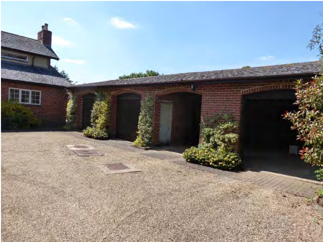
Plate 4: Sycamore Lodge garages, viewed from the parking area
