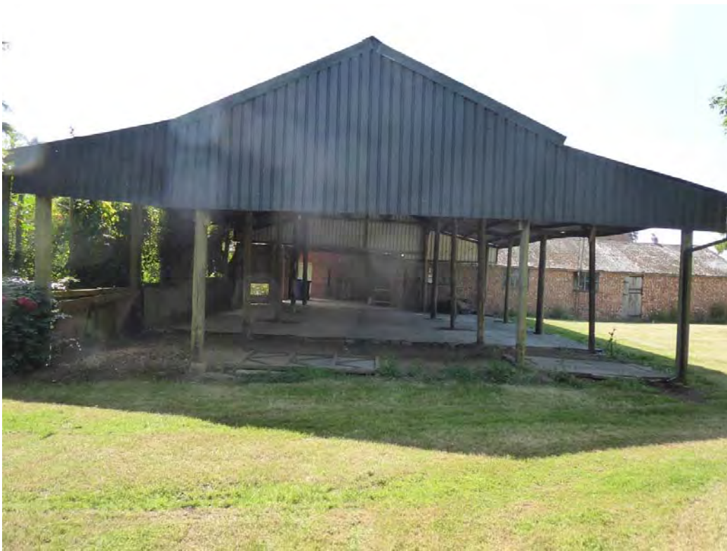
Plate 5: Steel roofed shelter and brick and asbestos roofed barn/byres
