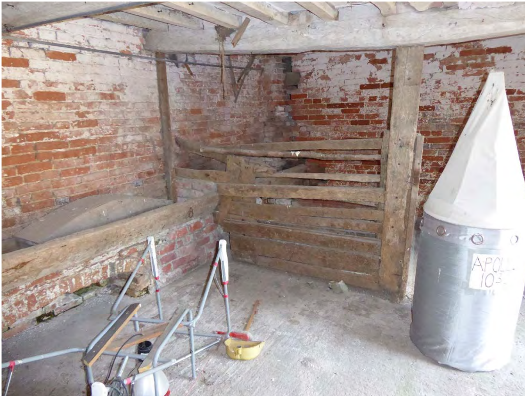
Plate 14: Interior of single storey byres
