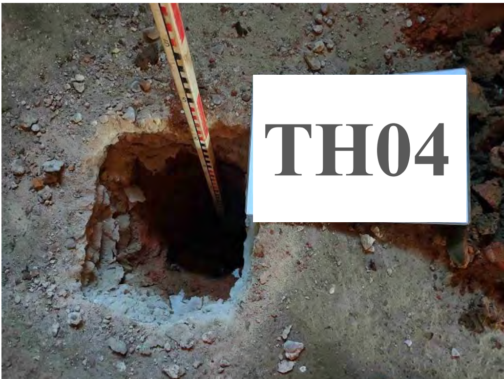
Plate 12: Trial hole TH04 on completion
