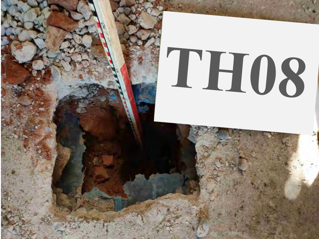
Plate 19: Trial hole TH08 on completion
