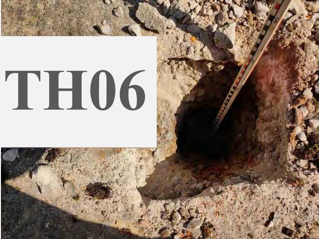
Plate 15: Trial hole TH06 on completion
