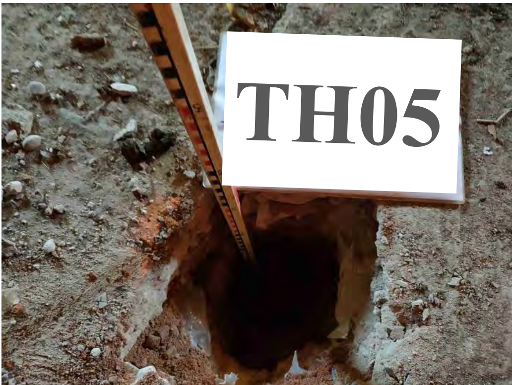
Plate 14: Trial hole TH05 on completion
