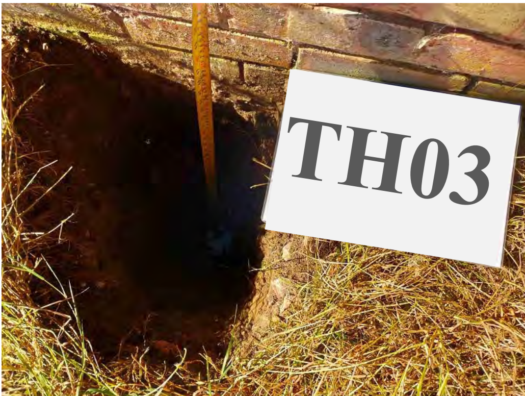
Plate 10: Trial hole TH03 on completion
