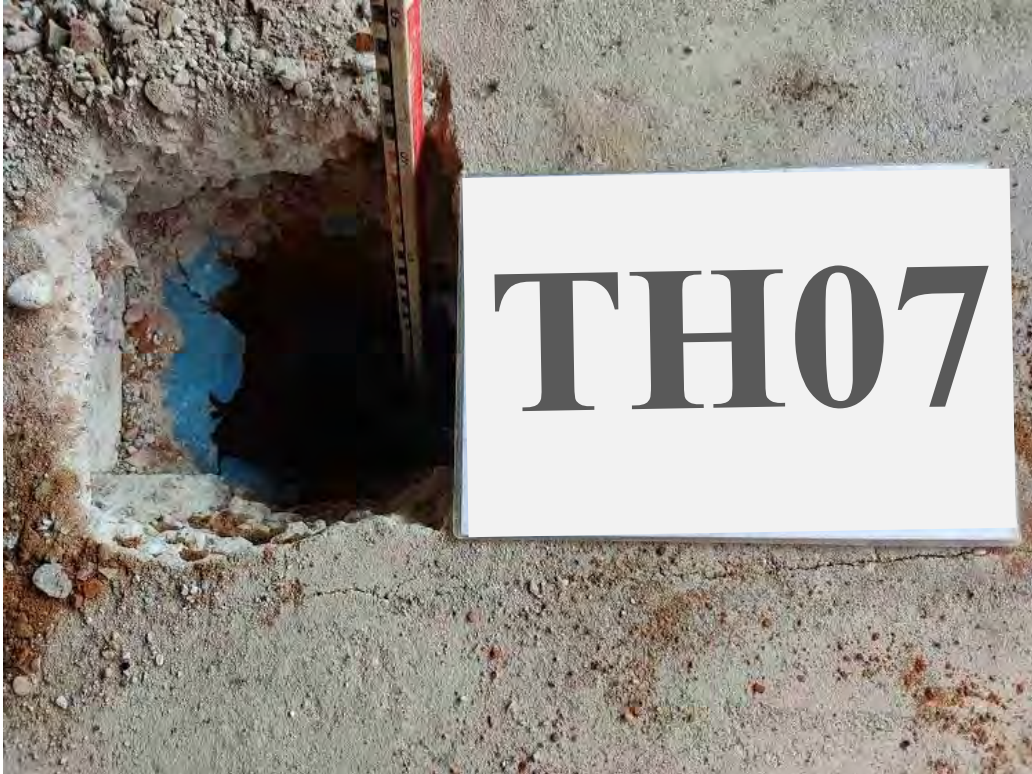
Plate 17: Trial hole TH07 on completion
