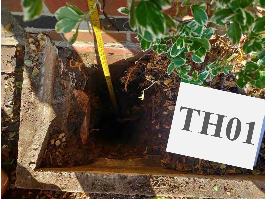
Plate 7: Trial hole TH01 on completion
