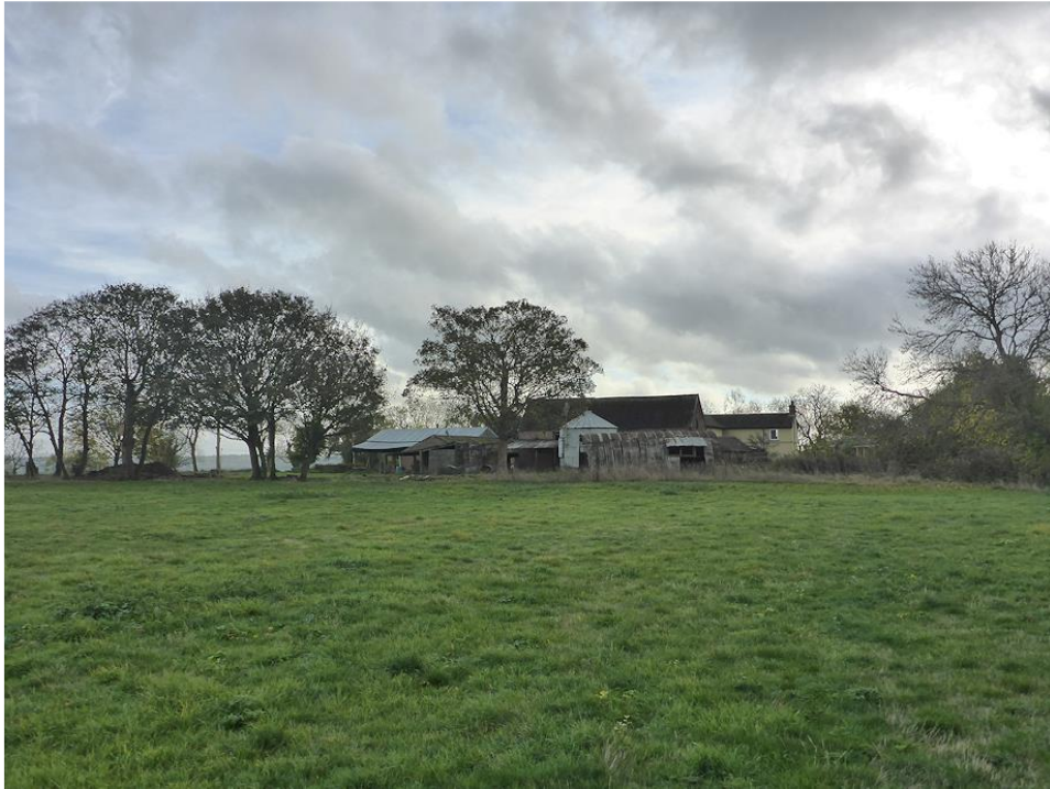
The rear of the property looking southeast.
