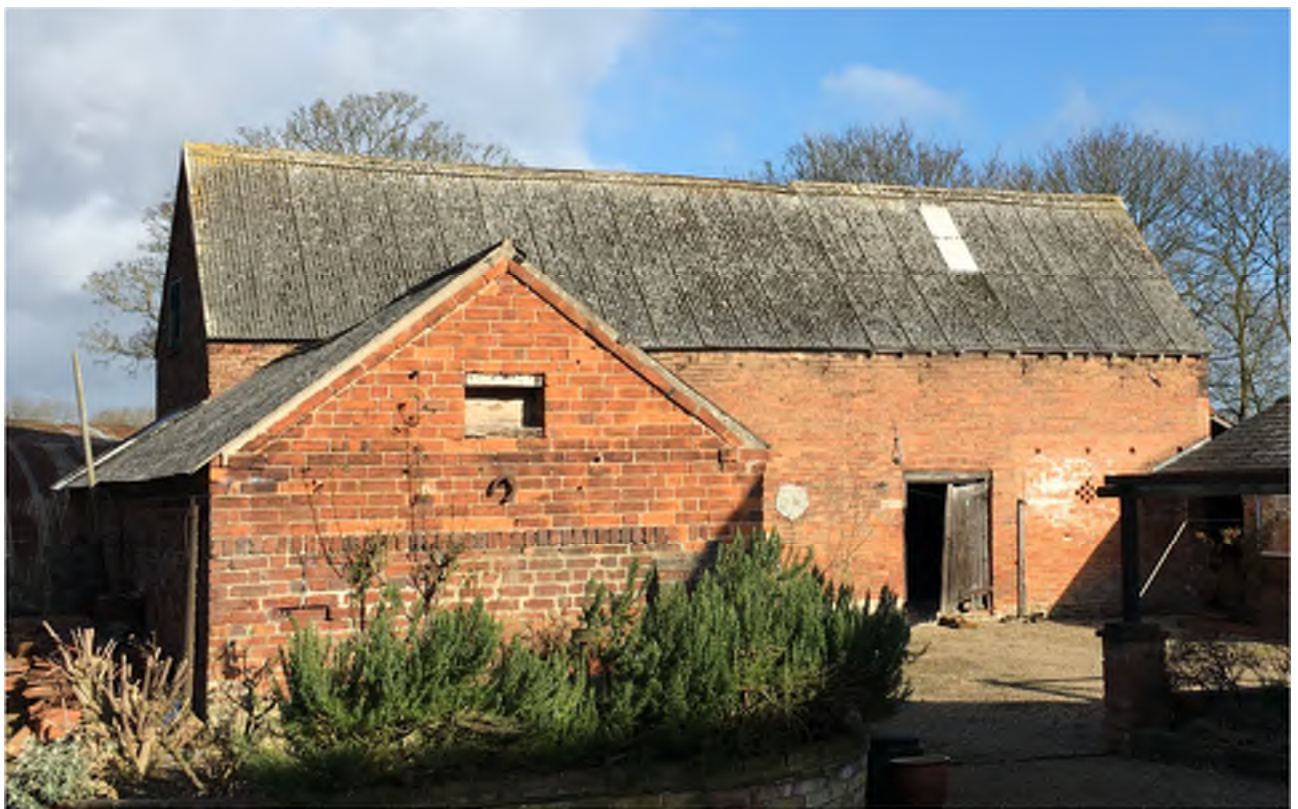
Stables in foreground, Threshing Barn beyond
