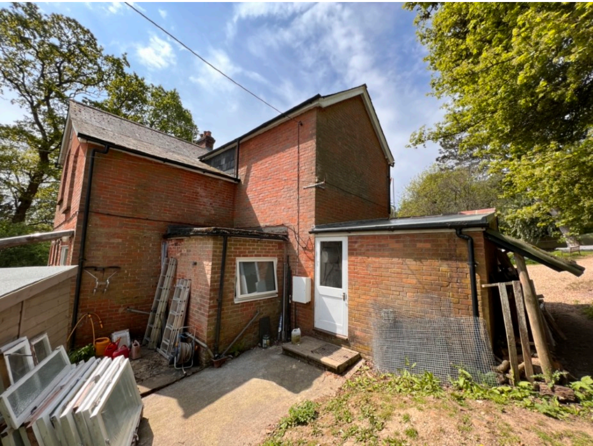
Fig. 7. View from boundary towards side (north) elevation
