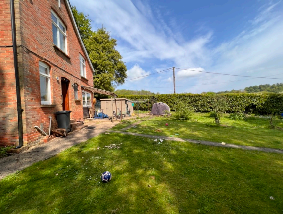
Fig. 4. Rear elevation, view towards boundary with Snode Hill road
