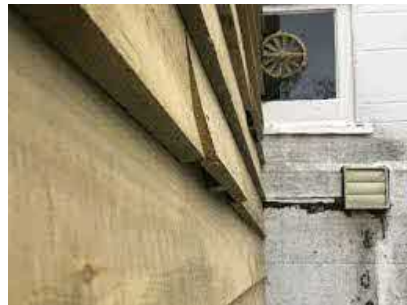
Figure 10 – Pegged cladding technique
