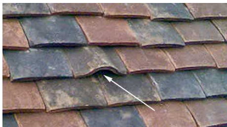
Figure 7 – ‘Tudor’ Bat access tiles
