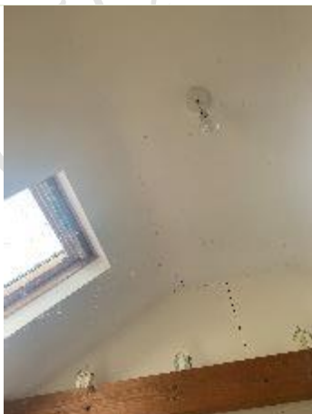
The vaulted ceiling – there is no loft void
