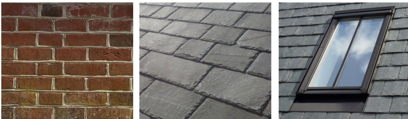
Figures 16-18. Example materials - Brickwork, slate roof tiles, conservation rooflights.
