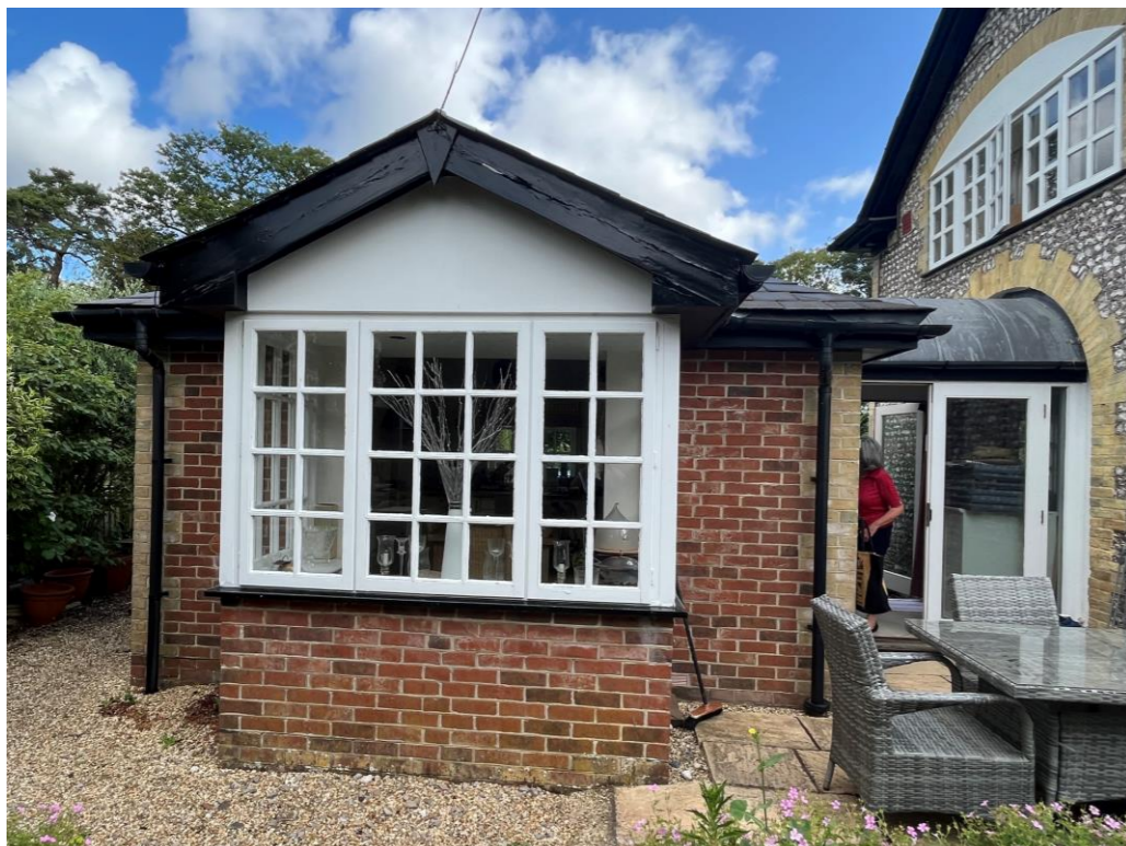
Figure 10. Rear of brickwork kitchen extension and glazed entrance space.
