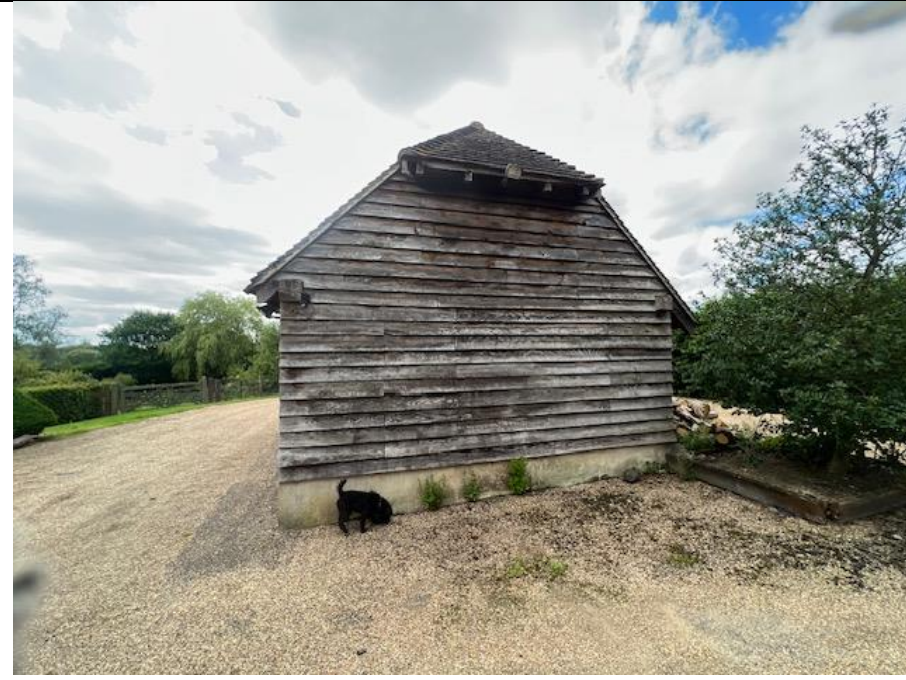
PHOTOGRAPH 15: East facing elevation of the Garage showing the weather boarding.
