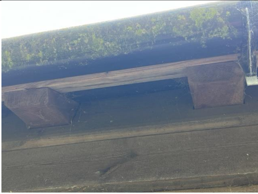
PHOTOGRAPH 11: The eaves of the Annex and Gym are sealed.
