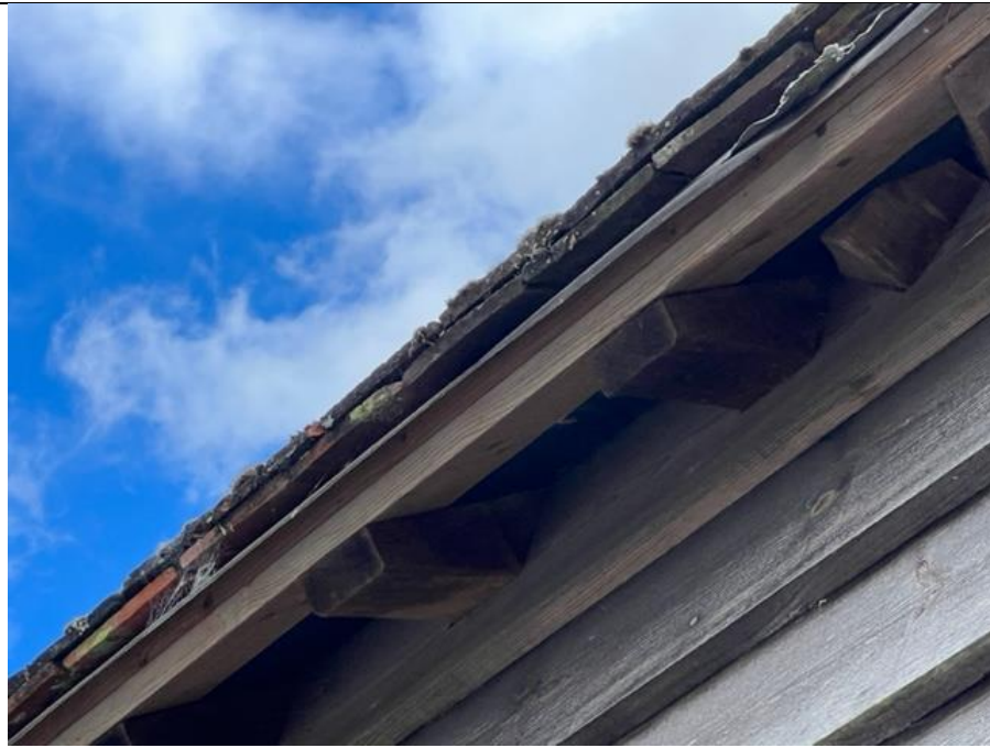
PHOTOGRAPH 18: The eaves are sealed throughout the Garage and Workshop.
