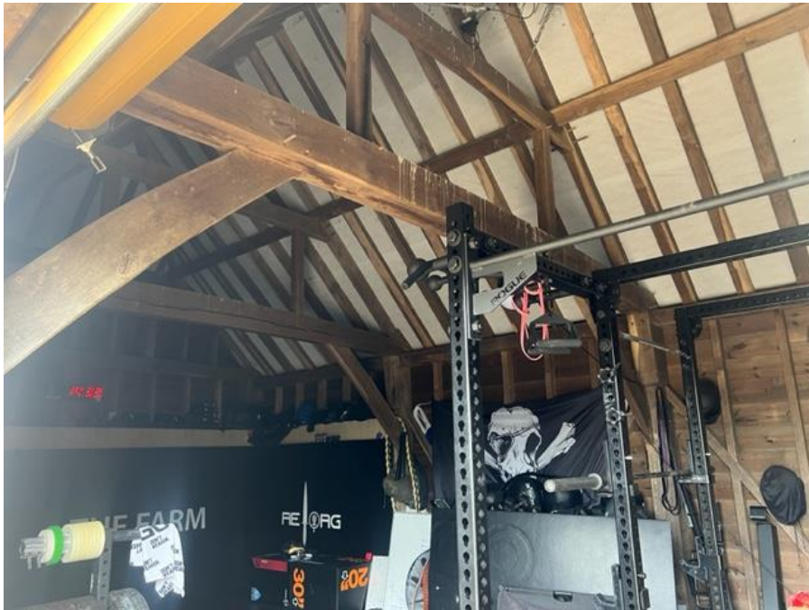
PHOTOGRAPH 6: Internally the Gym is single skinned and has a roofing membrane beneath the tiles.
