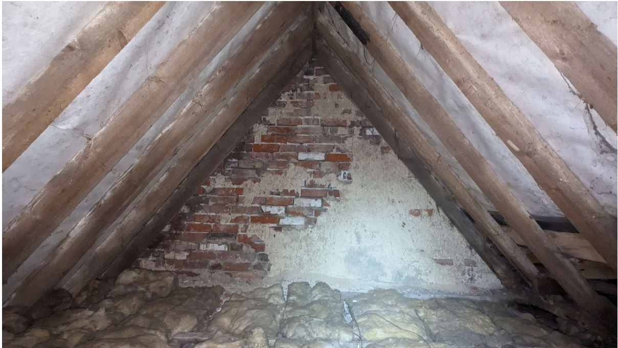
Photo 4 – View inside the loft space.
