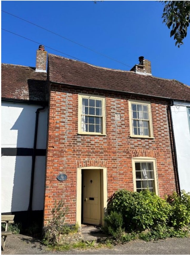
1. West (principal) elevation of Rosemary cottage.
