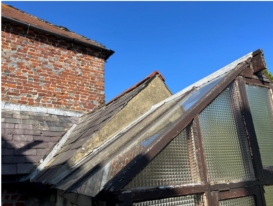
4. South elevation of existing single storey extension.
