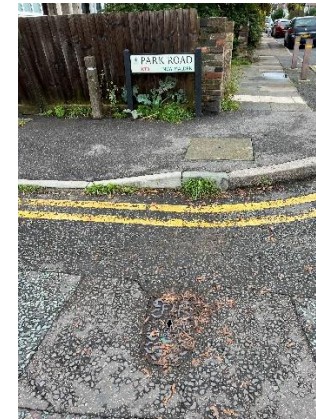
Fire hydrant at junction of Westbury Road and Park Road.
