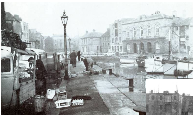
Fig 4: 1950s view of Quay Road & Sutton Harbour showing commercial uses established along the Quayside out of mini vans associated with the fishing industry. Taken prior to lock gates installed – water level dictated by the tides.
