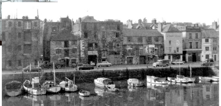
Fig 5: 1959 view of Quay Road & warehouses prior to redevelopment to restaurants/pub use. Shows quayside used for vehicular access & smaller fishing vessels moored up to quay.
