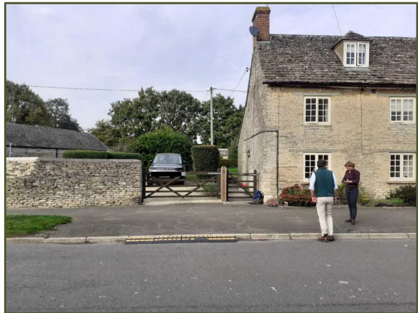
No.4 Park Street with parking area
