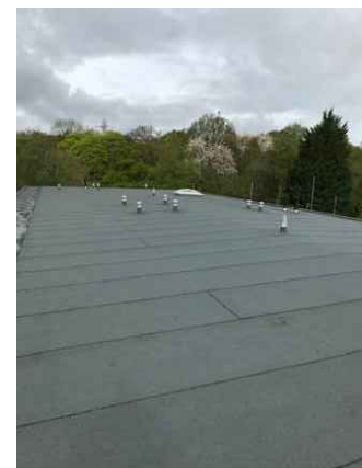
Roof Finish Polymer bitumen vented system for insulated 'warm roof' construction Colour - mid grey
