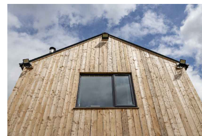
Wall Finish UK-sourced, sustainable larch cladding (panels approx. 120mm wide) Colour - natural timber
