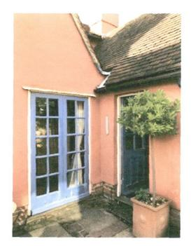
Proposed pitched roof veranda over backdoor and French doors in area shown. Oak framed, single oak post at outer corner, glass roof, lead flashings. Lead box gutter to replace existing plastic gutter above backdoor discharging to cast collector and downpipe replacing existing plastic items
