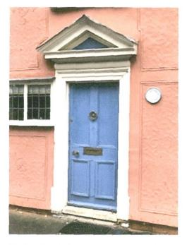
Timber front door beyond repair. To be replaced on a like for like basis in timber reusing all existing door furniture.
