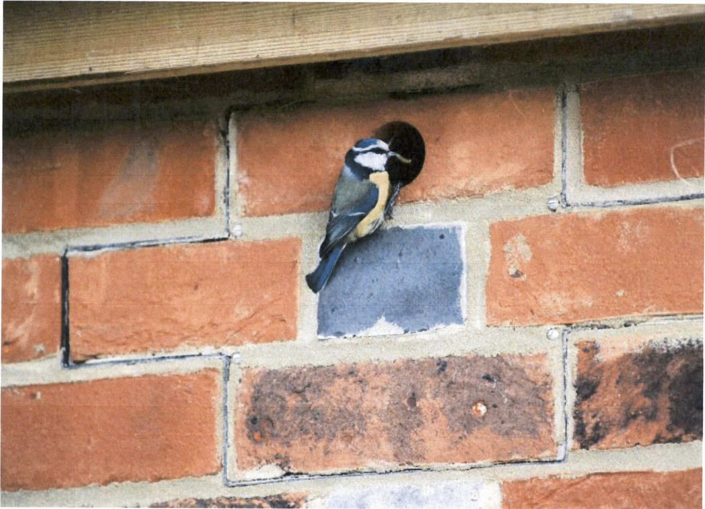
Blue tit using a Standard bird box; not fully mortared in, allowing box front to be removed for cleaning and monitoring
