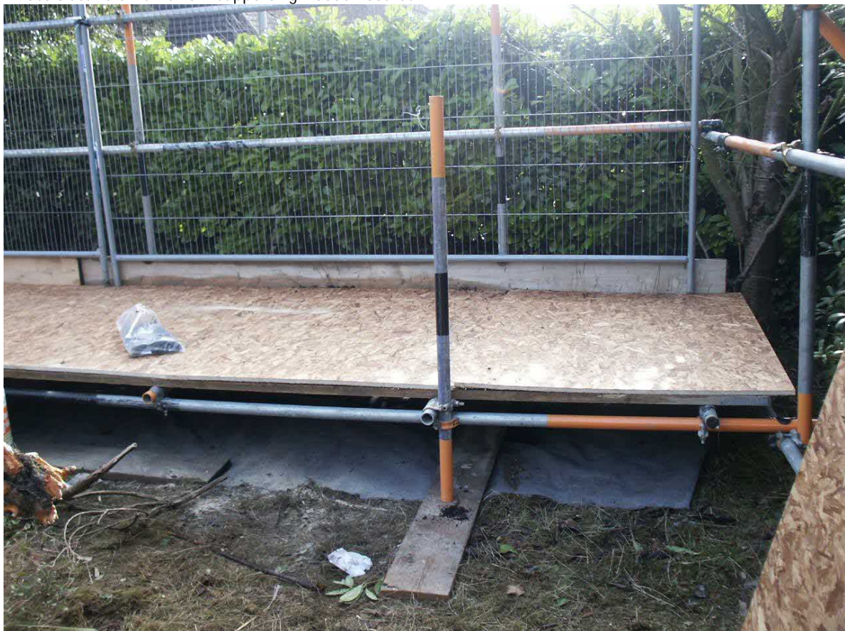
Photo 3 Scaffold framework supporting wooden boards
