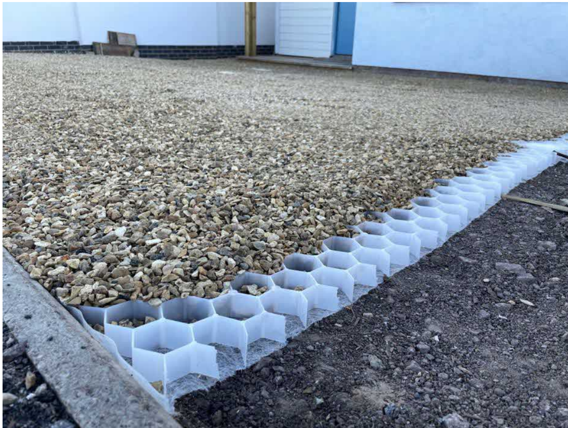
Photo 1 An example of a gravel grid driveway under construction
