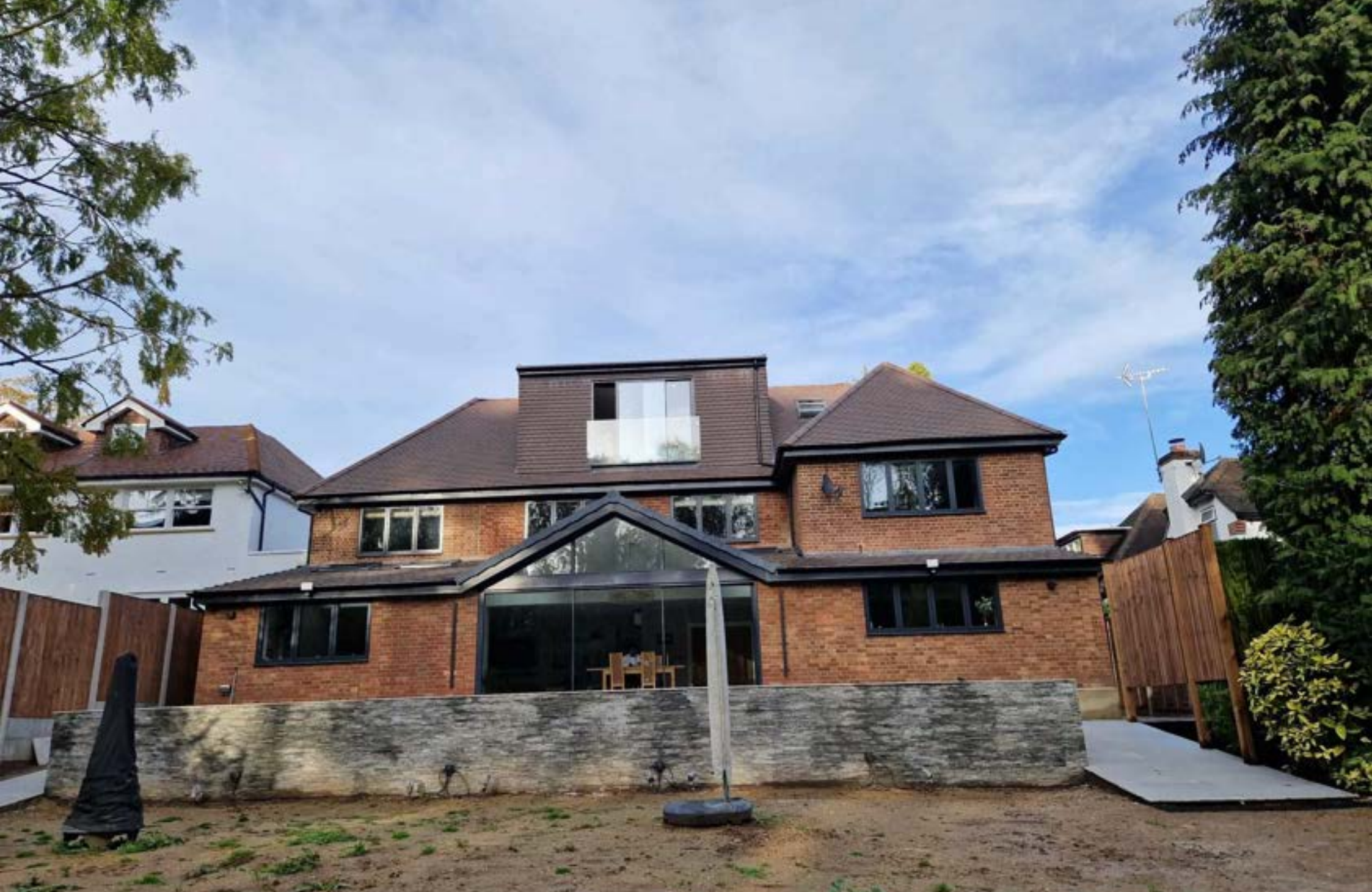
REAR VIEW OF COMPLETED EXTENSION AND PATIO
