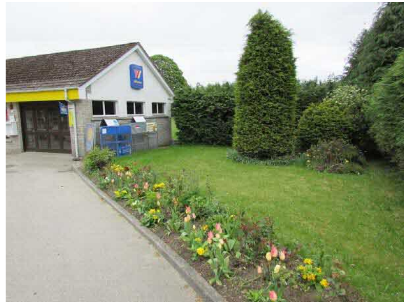
Three fuel dispensing pumps on the forecourt with no sign of staining
